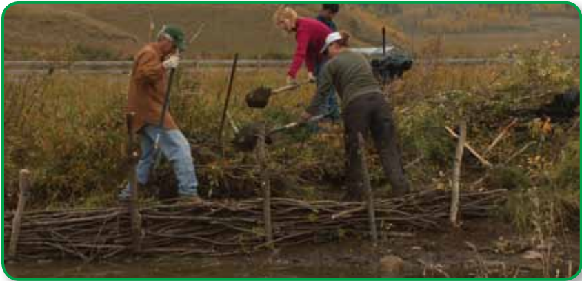
Bioengineered wattle fence.
