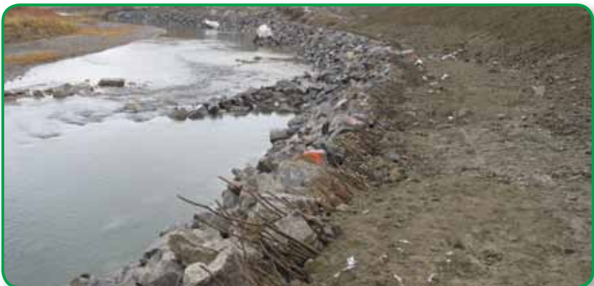
Biotechnical stone toe protection with brush layering.
