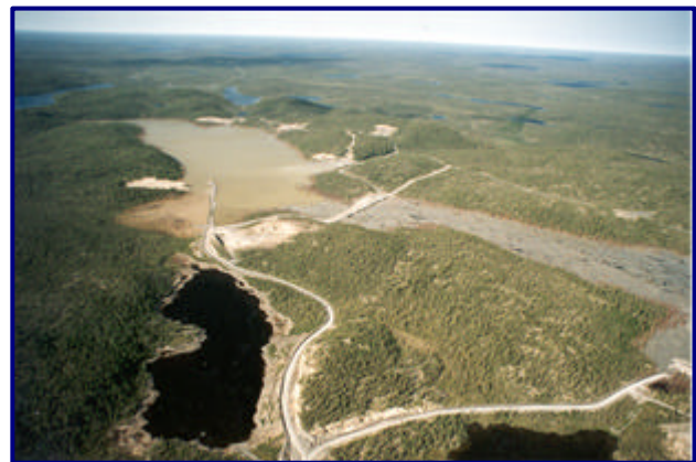
Tailings at Colomac Mine, NWT
