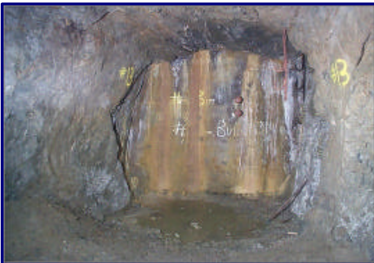
Bulkhead at Giant mine, NWT
