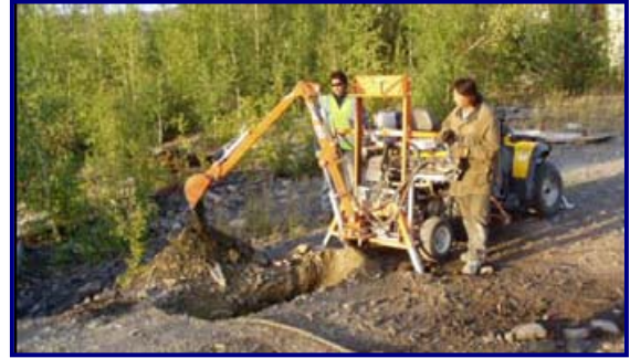
Excavating contaminated soil at Discovery
