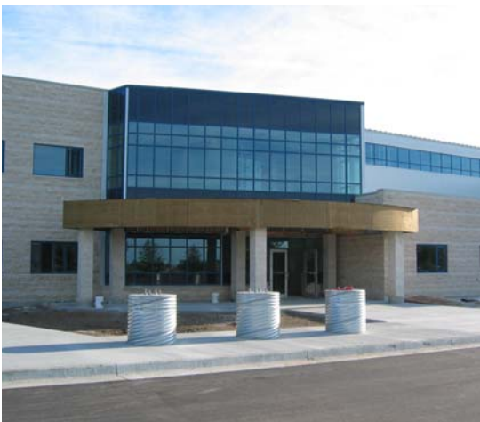
DCC's innovative approach to the 2 PPCLI design-build contract helped ensure the unit's new CFB Shilo headquarter facility was completed on time.
