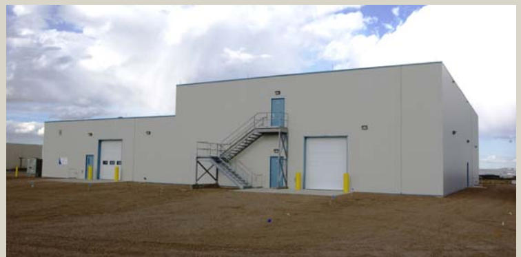
CFB Suffield's Indoor Training Arena features moveable wall panels to control the size and shape of various scenarios.
