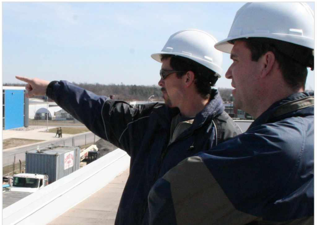
Dave Long, Contract Coordinator at DCC's Kingston site office (left) and Paul Ireland, Site Manager, survey a parking lot adjacent to the Theatre Activation Team (TAT) Warehouse project, currently under construction.
