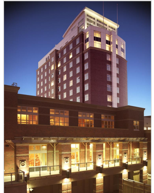
The $32.5-million Juno Building at CFB Halifax was completed in May 2005. The project received the Canadian Design-Build Institute's 2006 Award of Excellence in September. The award provided well-deserved industry recognition for DND as the building's owner, PCL Constructors Canada Inc. as the principal contractor and WHW Architects as the design consultant team.
