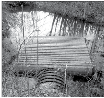
A baffle protect this culvert from beavers while letting fish through.
