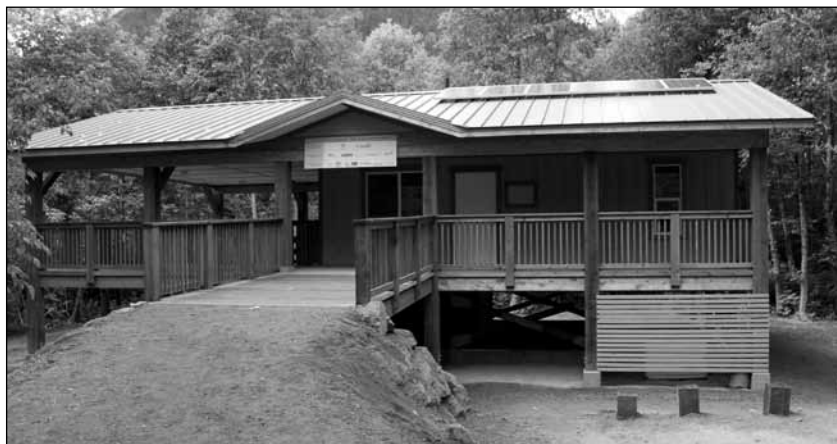
The building is completely off-grid, featuring solar power, composting toilets and rainwater catchment. Photo: Veronica Woodruff.
