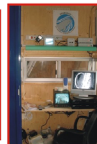
Sound generating & recording equipment in equipment cabin
