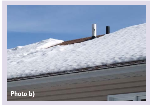
Examples of sub-slab depressurization system with a roof exhaust stack a) Ice build-up on a un-insulated system b) Insulated system with fan in the attic
