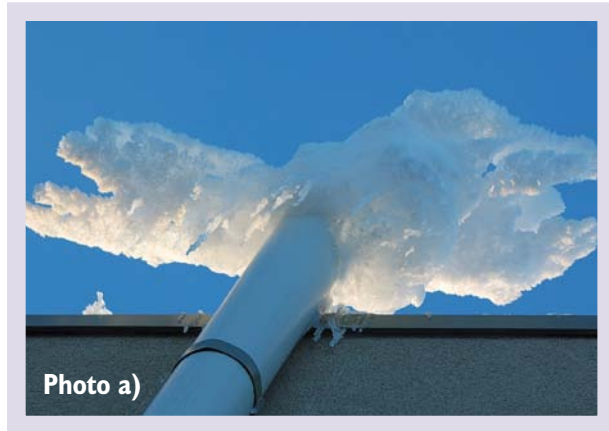
Examples of sub-slab depressurization system with a roof exhaust stack a) Ice build-up on a un-insulated system b) Insulated system with fan in the attic
