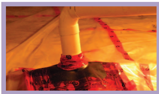
Photo 5 – Sealing the penetration through the membrane
