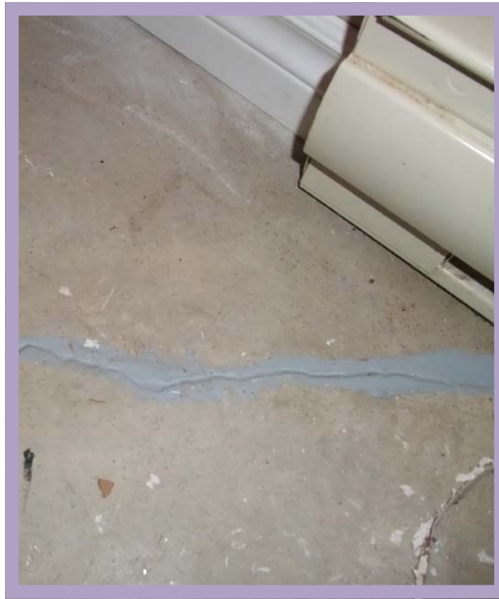
Photo 8 – Sealed Crack in Concrete Slab
