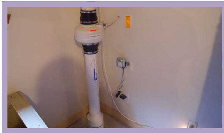
Photo 3 – Basement Fan Installation
