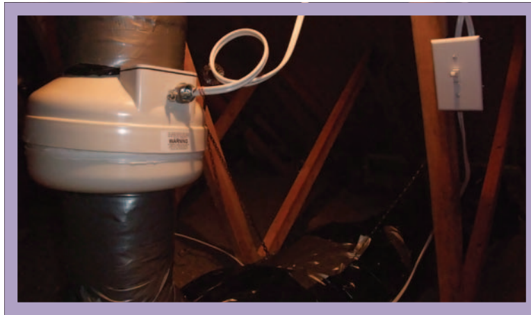
Photo 2 – Attic Fan Installation
