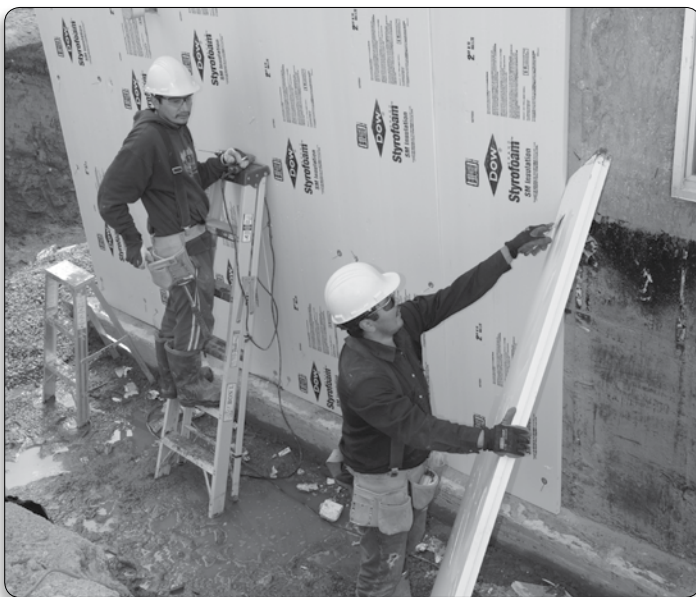
Insulate foundation walls
