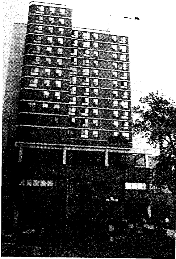
Figure 1: View from the street
