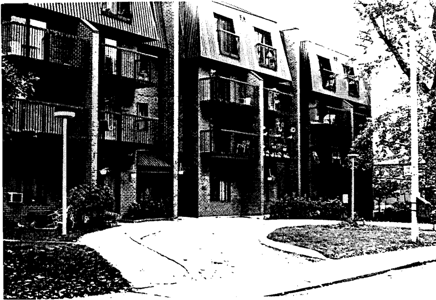
Figure 22: View from the street
