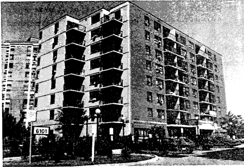
Figure 15: View from the street
