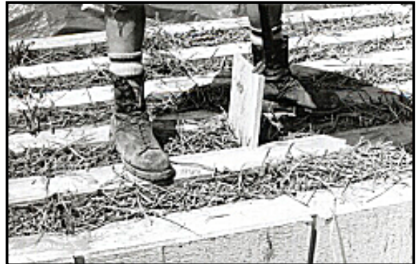
Fig. 3.4.2-2 Block dividers being removed from formwork
