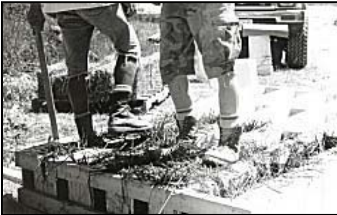
Fig. 3.4-1 Straw clay mix is lightly tamped into forms
