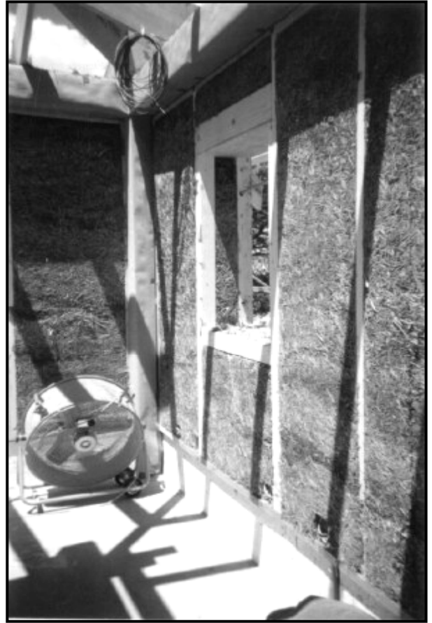
Fig. 1.2-3 Completely formed wall
