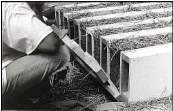
Fig. 3.4.2-3 Removal of block width keys
