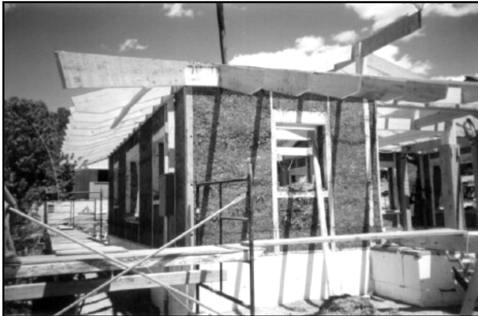
Fig. 1.2-4 Exterior view of walls prior to plastering
