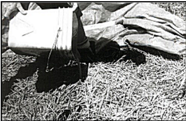
Fig. 3.3-1 Clay slurry being broadcast over straw.
