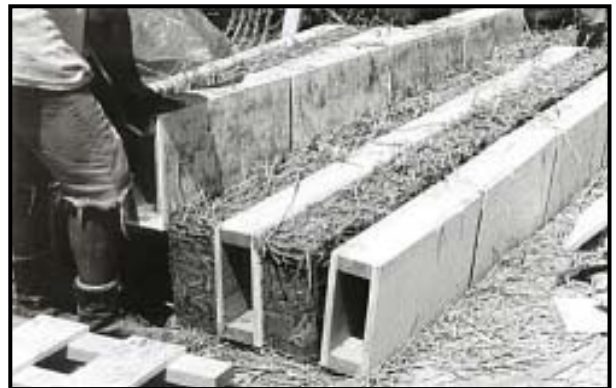
Fig. 3.4.2-4 Screeding effect of form walls.
