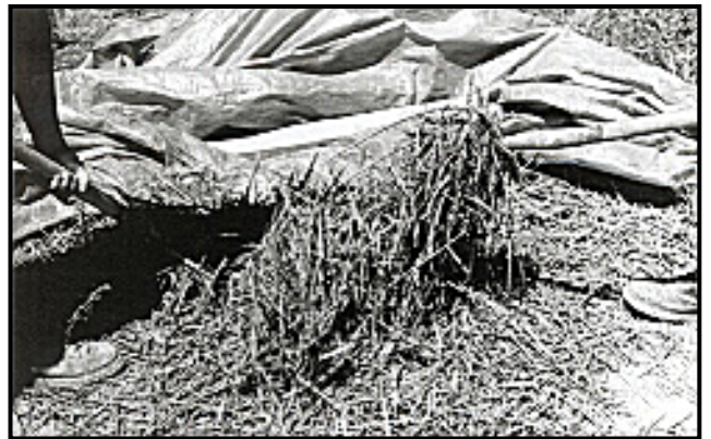
Fig.3.3-2 Straw being mixed with slurry
