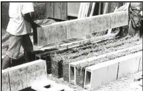
Fig. 3.4.2-5 Removal of form walls
