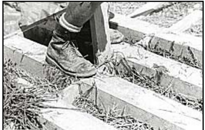
Fig. 3.4-2 Straw clay being tamped with 2x4 around edges of form
