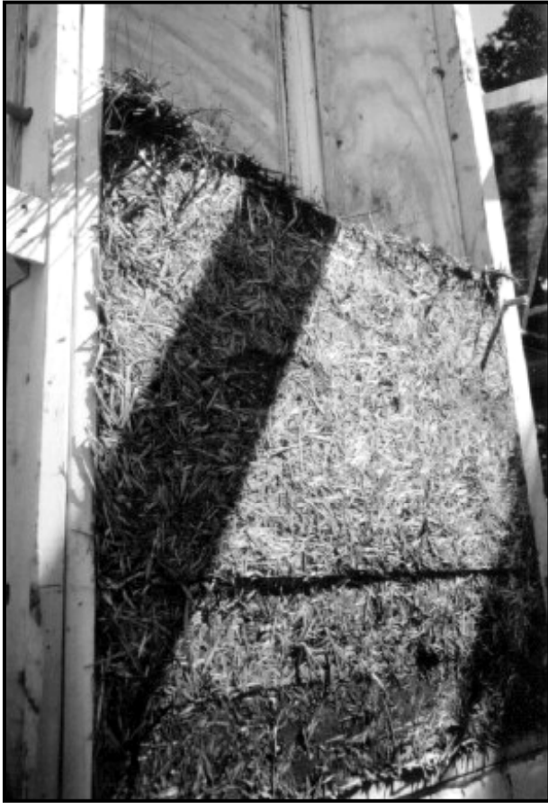
Fig. 1.2-2 View of wall upon removal of first tier of formwork.
