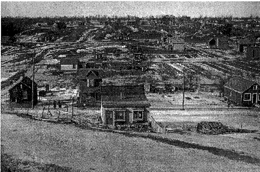
Photo 5: Earlscourt under Development, Toronto (circa 1916)
