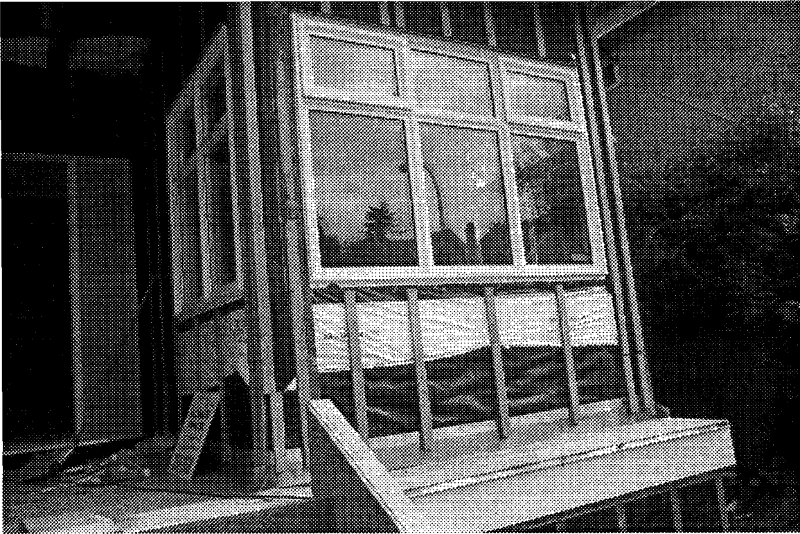
Triplex south elevation showing close up of vertical strapping around windows
