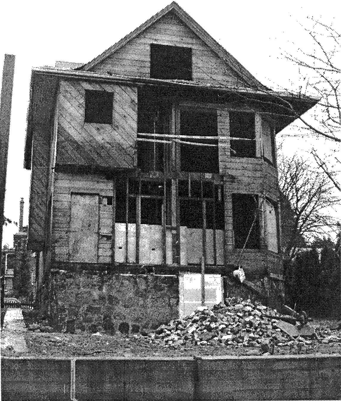
Triplex north elevation stripped to sheathing and framing, original stone foundation
