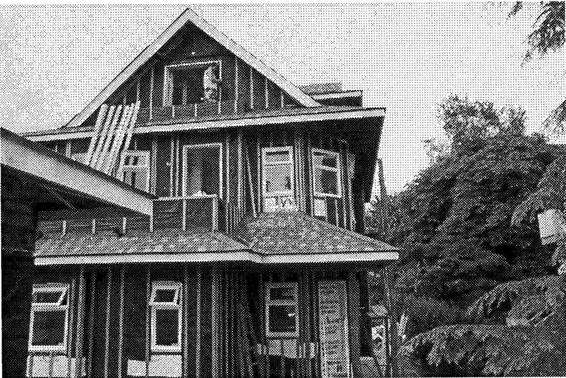
North elevation showing building paper and vertical strapping for rain screen wall cavity
