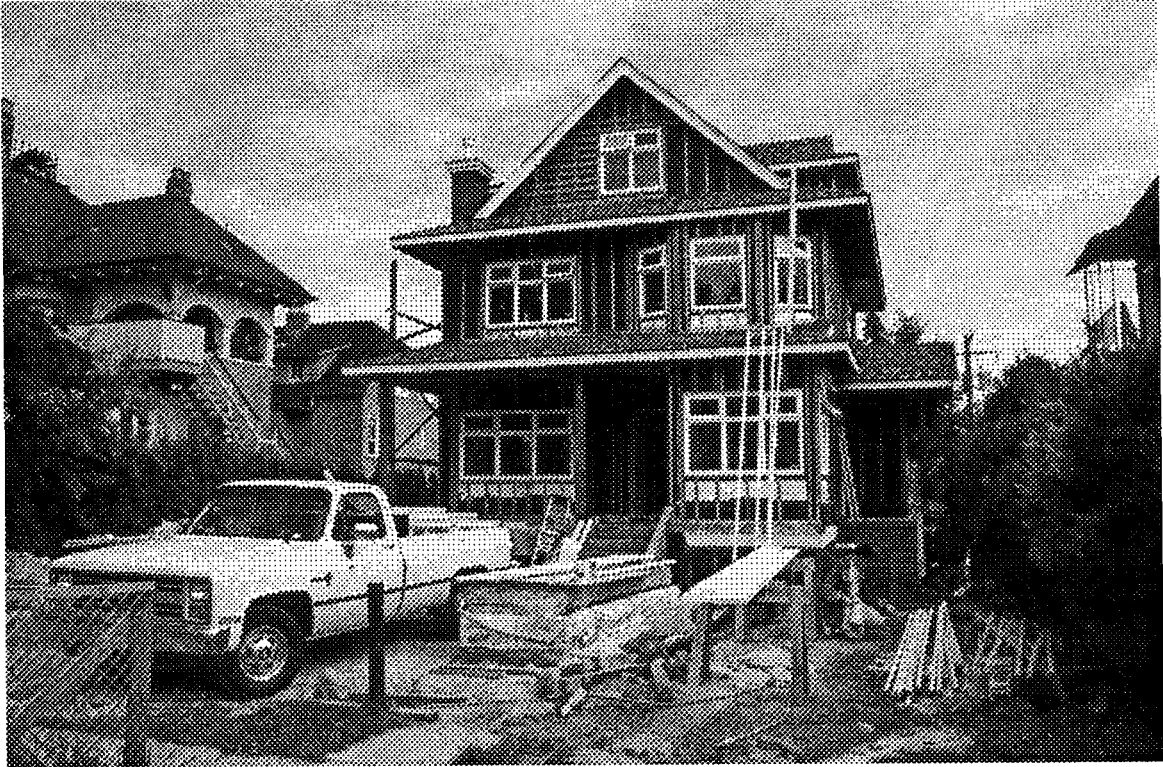
South elevation triplex showing building paper and vertical strapping for rain screen wall cavity
