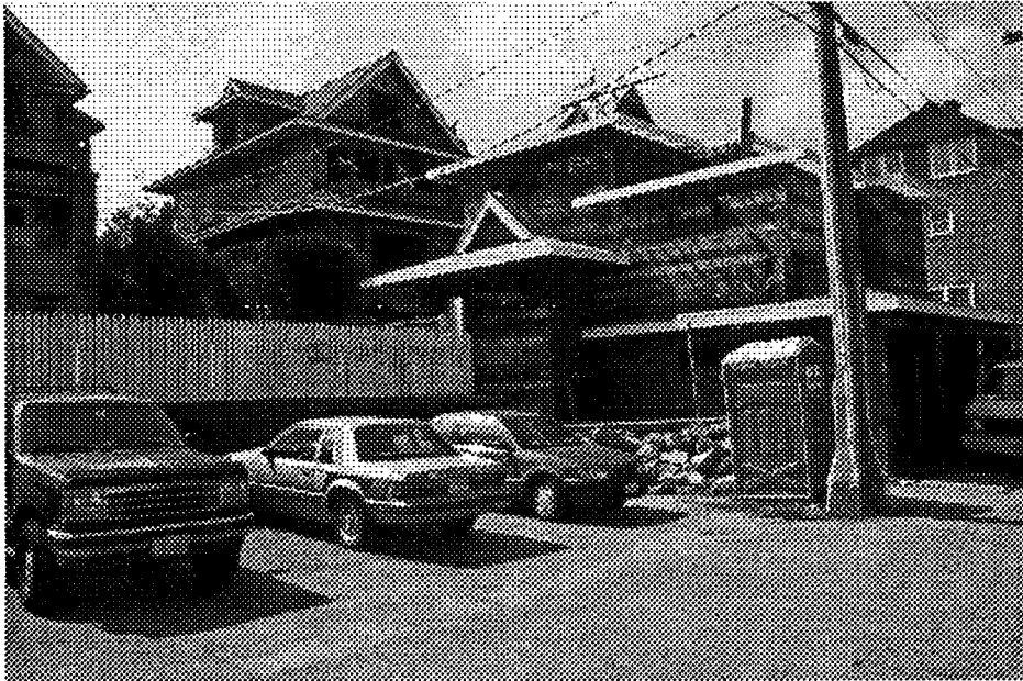
Coach house and rear of triplex shown from alley during framing
