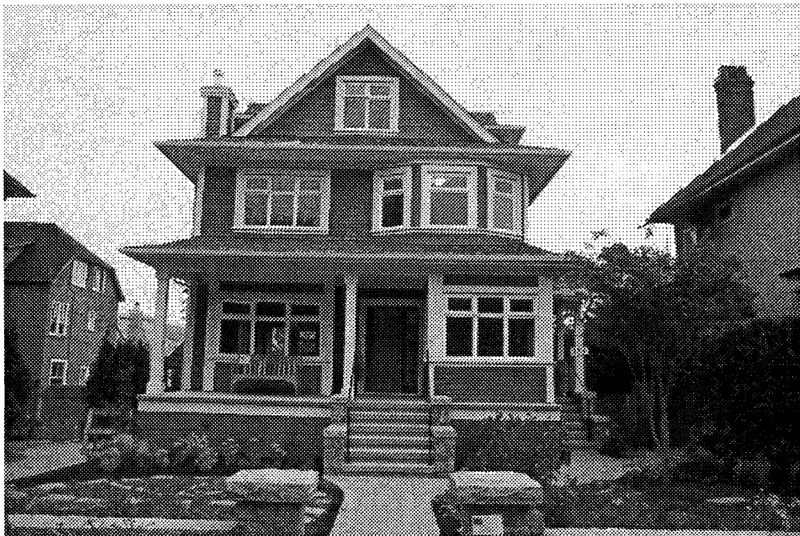
Finished triplex south elevation
