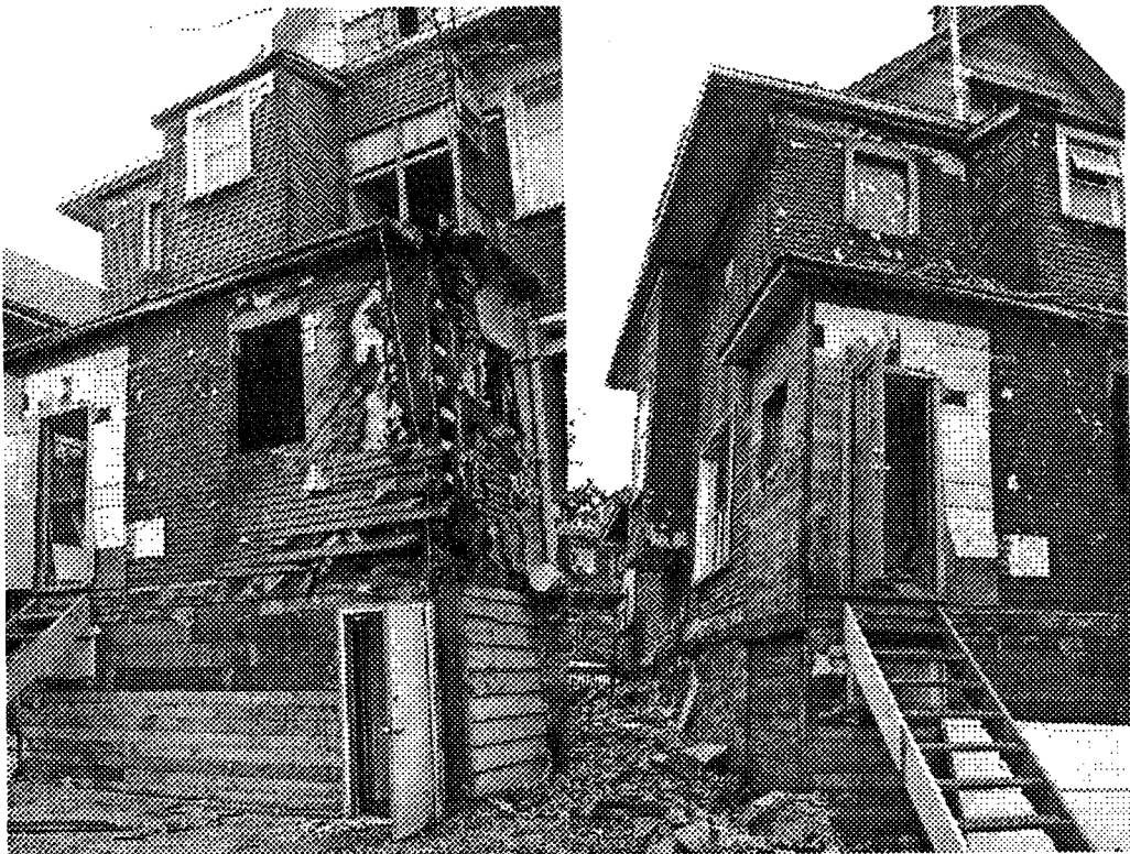
Original siding being stripped from triplex south and north elevations
