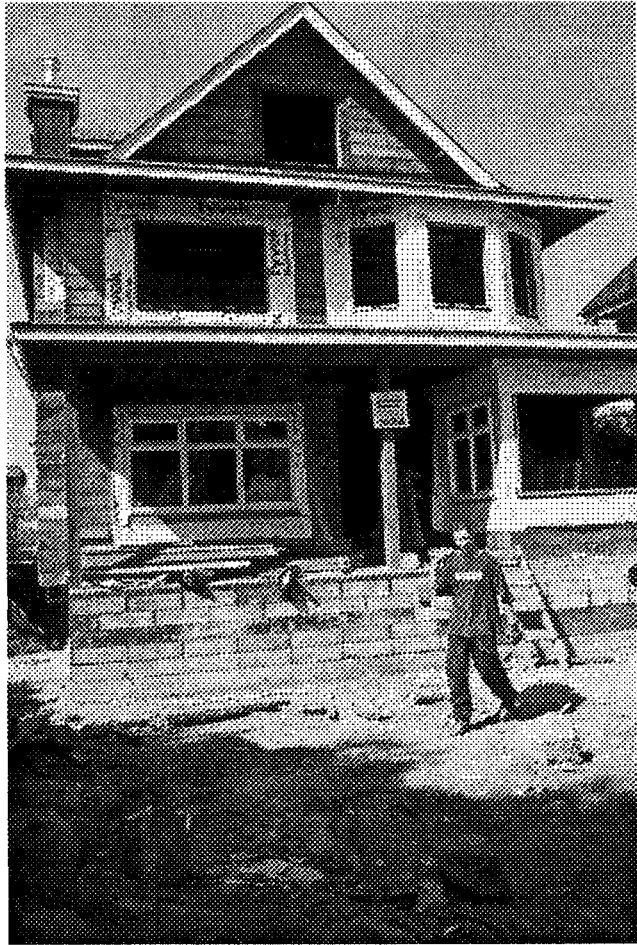
Triplex units showing sheathing and house wrap during window installation
