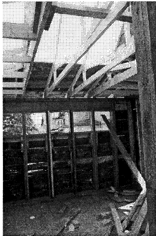
Coach house showing roof trusses and walls framed with salvaged lumber
