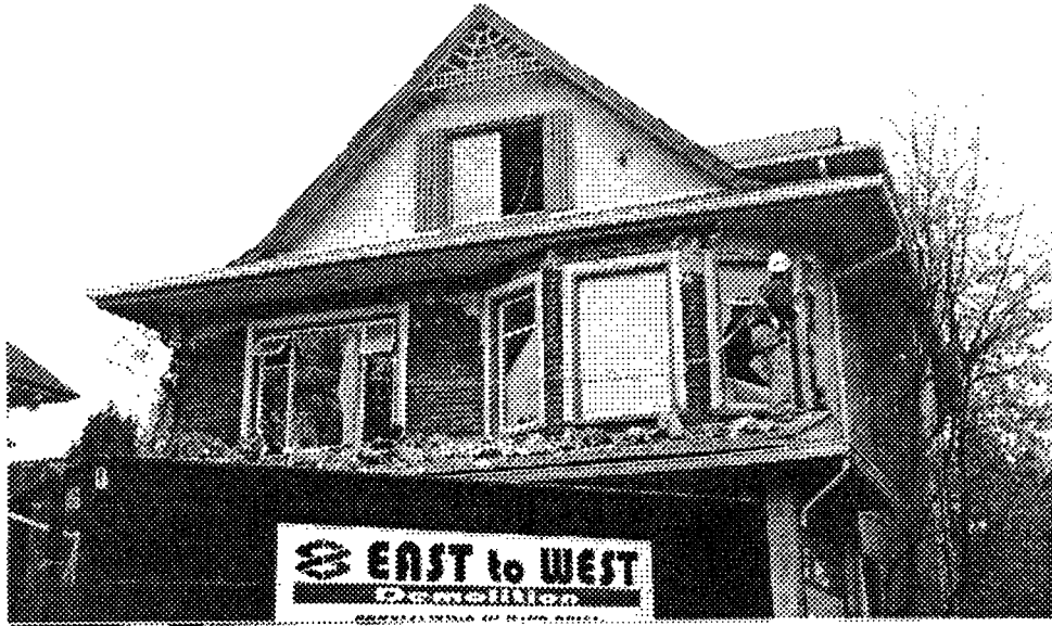
Stucco being stripped from triplex south elevation
