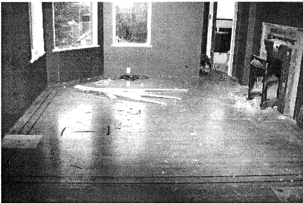
Interior main floor living room prior to development
