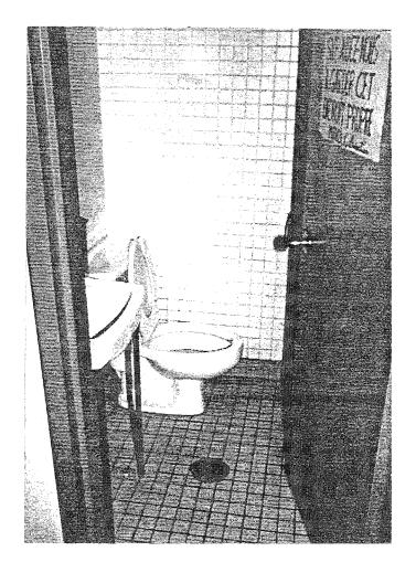
The clientele in low-income singles houses require more higher performing sanitary spaces as pertains to maintenance than those in family dwellings. The use of ceramic tile on all the floors and walls as well as a floor drain, making it possible to thoroughly wash down this space, is recommended.
