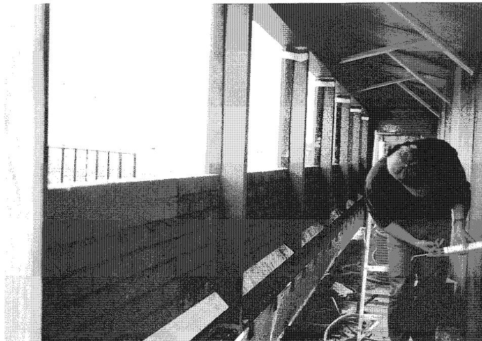
Photograph no.10: Erection of wall specimens.
