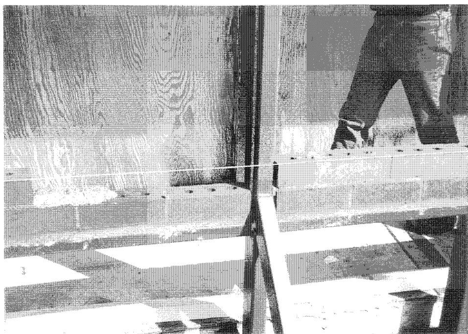
Photograph no.5: Erection and allignment of first two brick rows.
