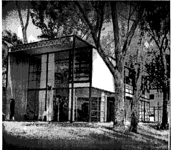
Figure 4: Modern Steel House
