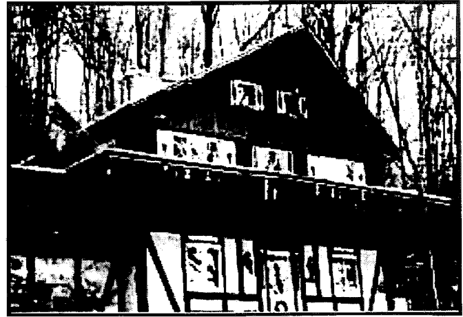
On a sunny day, this 110 sq.ft. SOLARWALL® heater, located in the gable, will raise the temperature of 150cfm of ventilation air about 50°F over ambient.
