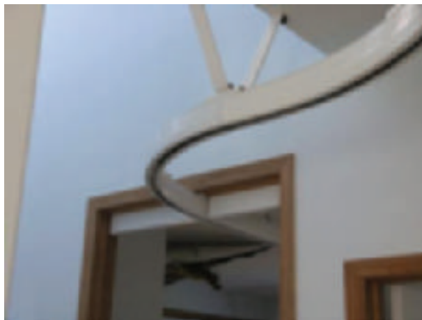
Figure 1—Doorway header renovation
