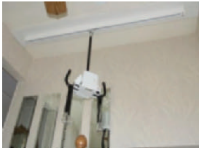
Figure 23 —ID#09 Ceiling lift used as an elevator
