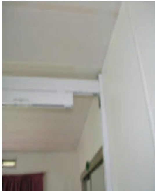
Figure 13—ID#04 Trailer home installation
