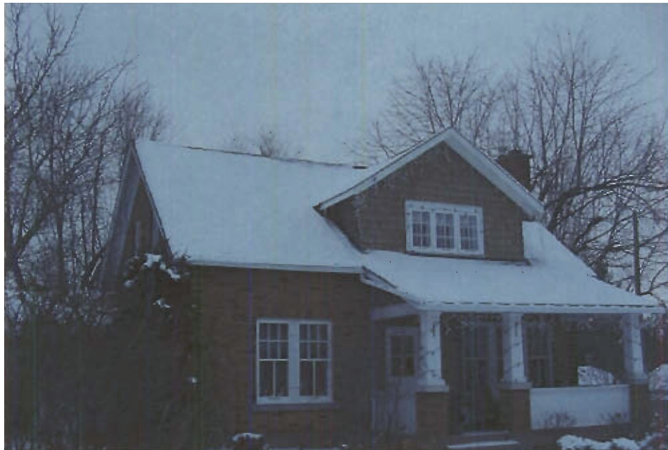
Photo 50: Manotick Single Family House
