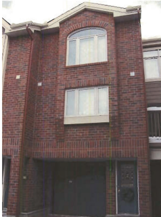
Photo 37: Site 3, Unrepaired Unit (front), January 20, 2004
