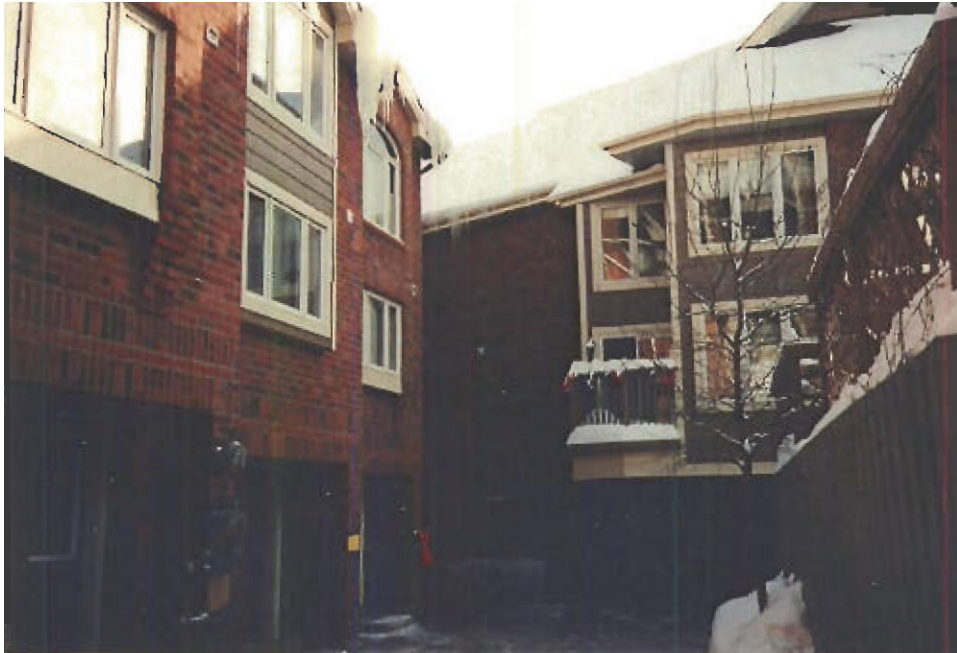
Photo 27: Site 3, Condominium Complex, Front Courtyard
