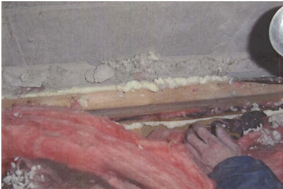
Photo 22: Site 2, Air Sealing Repairs at Party Wall
