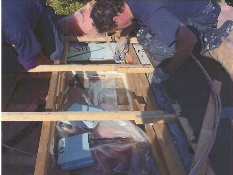
Photo 09: Site 1, Air Sealing Repairs, Party Wall in Cathedral Ceiling
