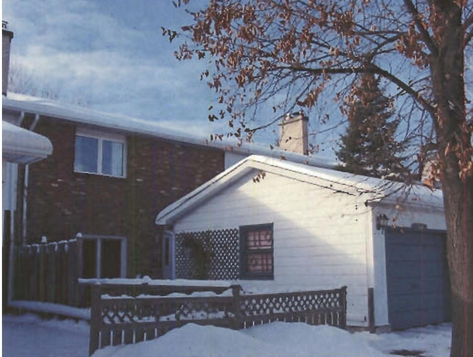
Photo 25: Site 2, Repaired Units, January 20, 2004
