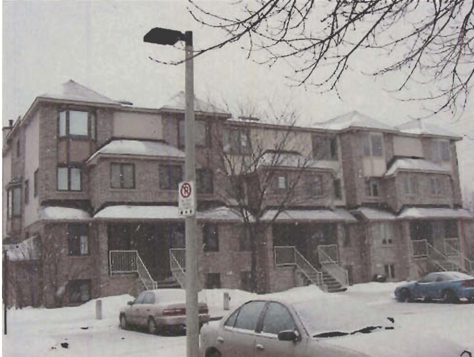
Photo 39: Site 4, Condominium Complex
