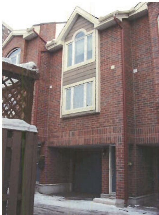
Photo 36: Site 3, Repaired Unit (front) January 20, 2004
