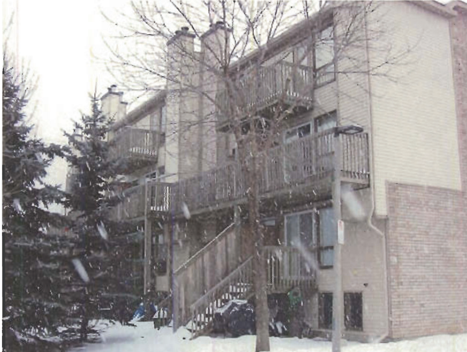
Photo 47: Site 4, Repaired Unit (back) January 20, 2004
