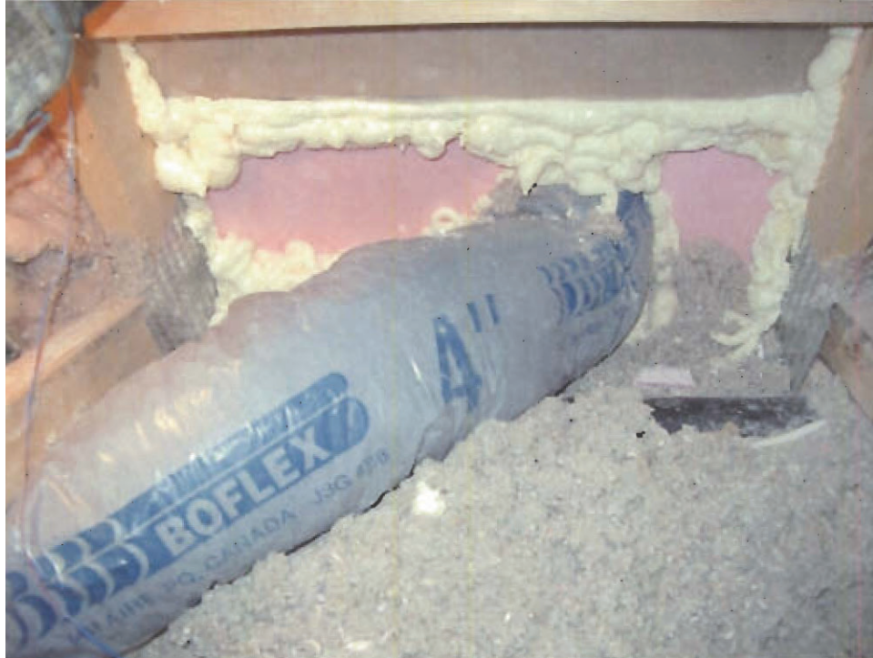
Photo 35: Site 3, Air Sealing
