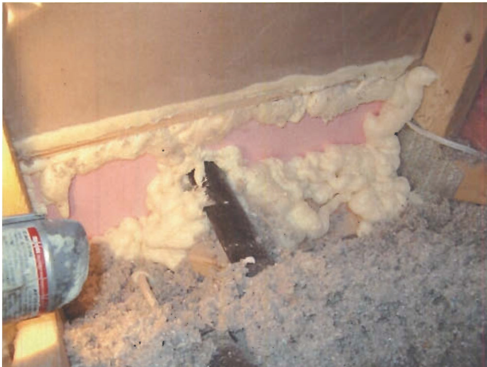
Photo 34: Site 3, Air Sealing
