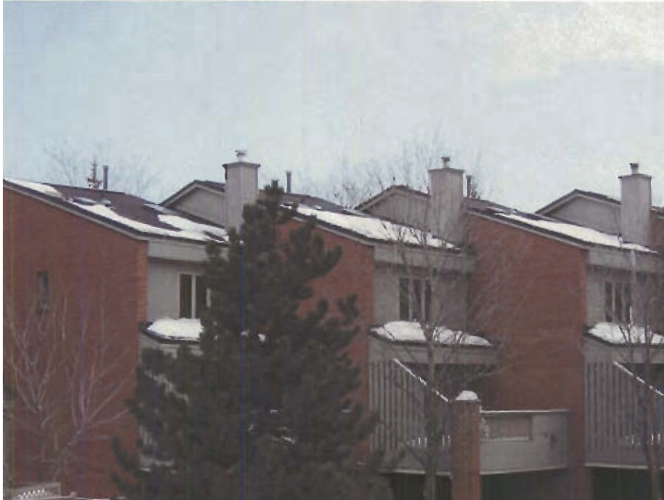
Photo 15: Site 1, Repaired Units, February 19, 2004
