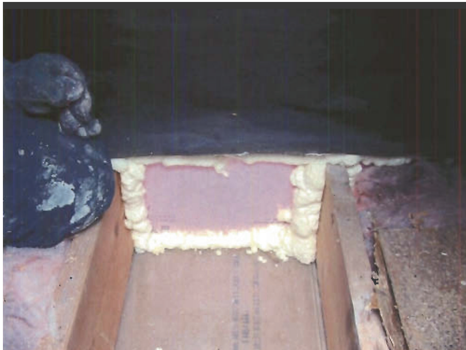
Photo 08: Site 1, Air Sealing Repairs, Joists
