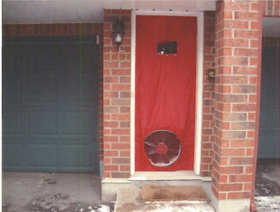
Photo 33: Site 3, Blower Door Installation
