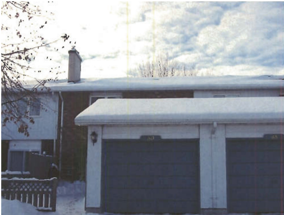
Photo 26: Site 2, Repaired Units, January 20, 2004
