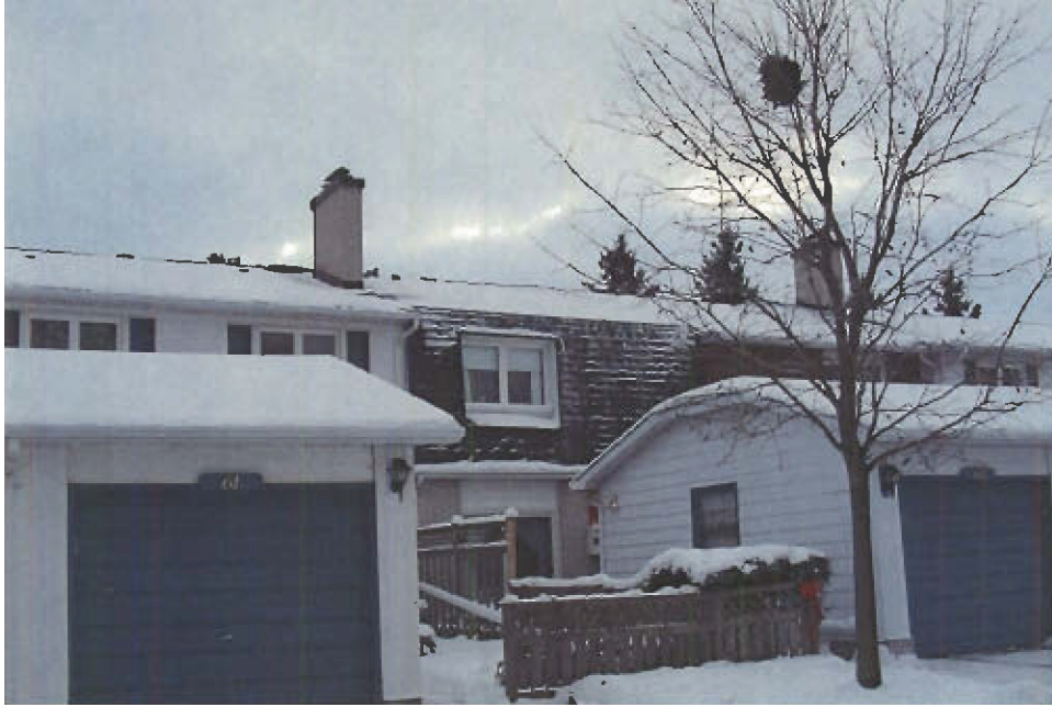
Photo 17: Site 2, Condominium Complex
