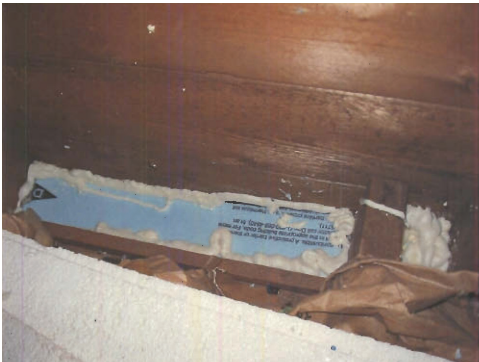
Photo 58: Manotick, Air Sealing of Balloon Framing Stud Space
