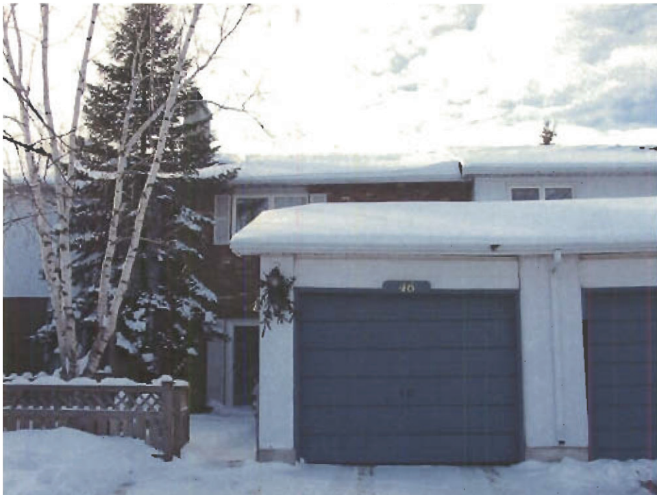
Photo 24: Site 2, Unrepaired Units, January 20, 2004
