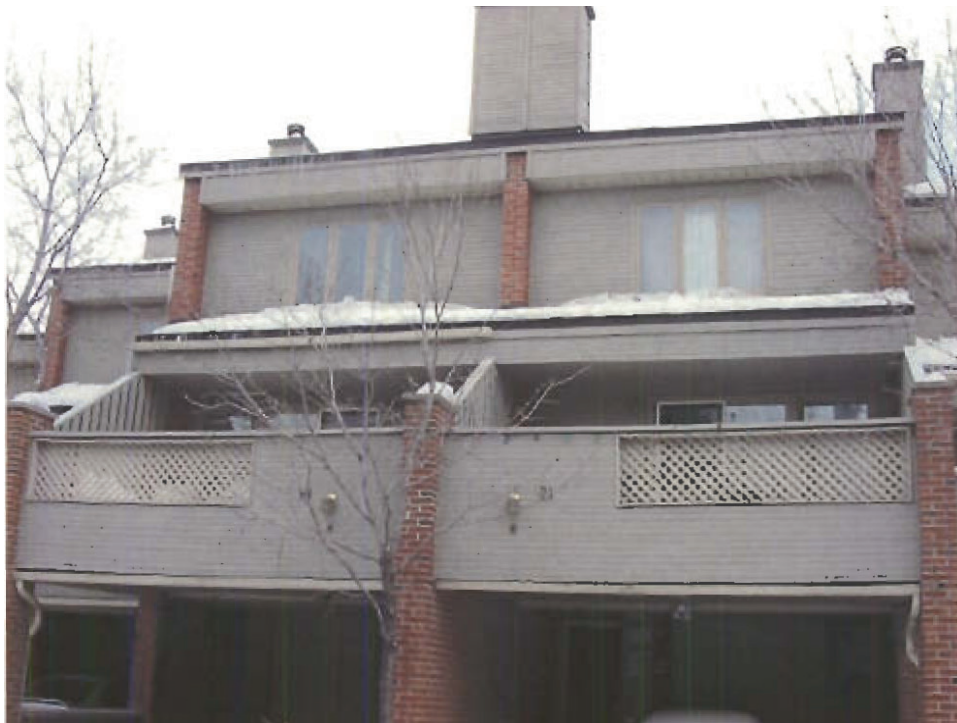
Photo 16: Site 1, Repaired Units, February 19, 2004
