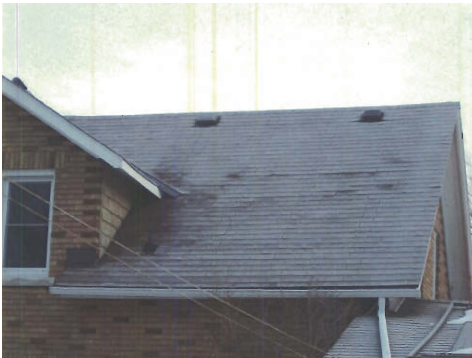
Photo 54: Manotick, Snow Melt Pattern (back of house)
