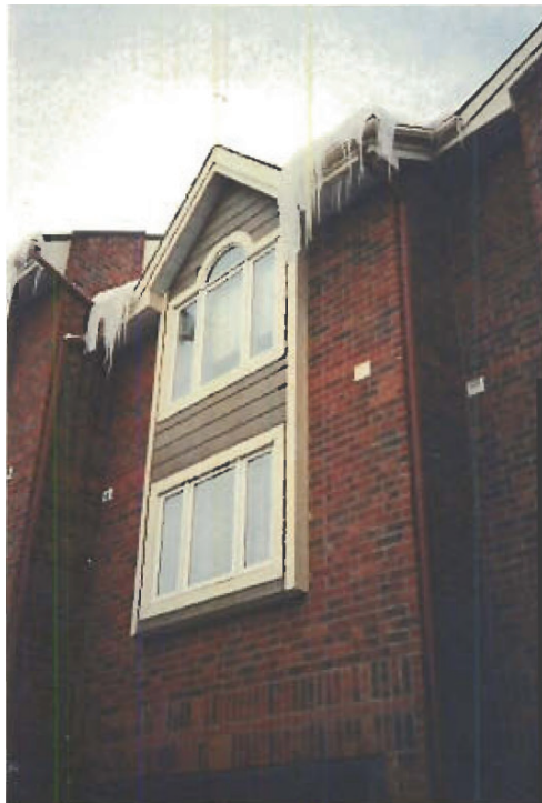
Photo 30: Site 3, Typical (past years) Ice Build-up
