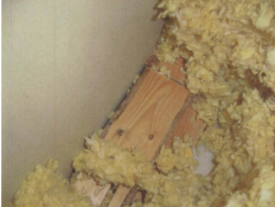
Photo 43: Site 4, Party Wall
