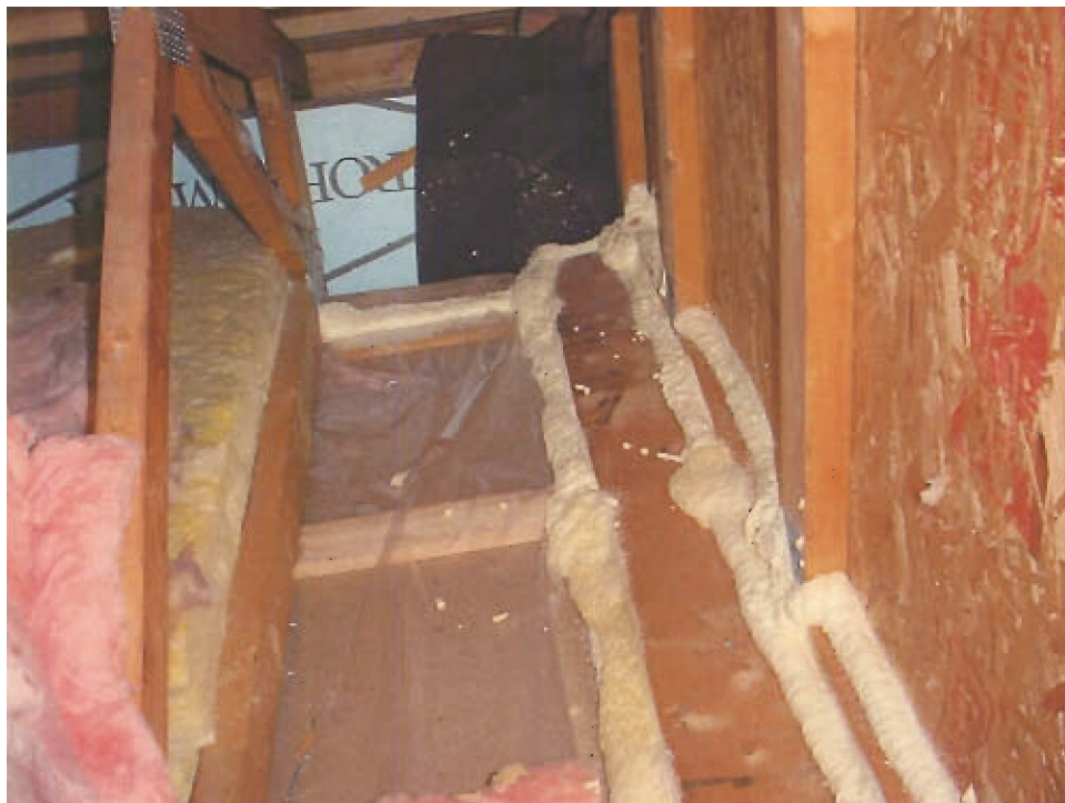
Photo 10: Site 1, Air Sealing Repairs, Party Wall in Main Attic
