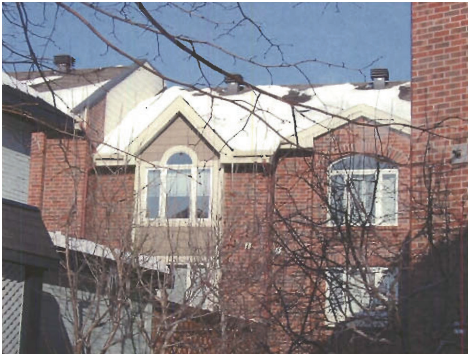
Photo 28: Site 3, Condominium Complex
