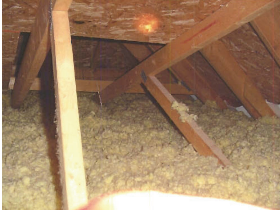
Photo 45: Site 4, New Baffles at Soffit
