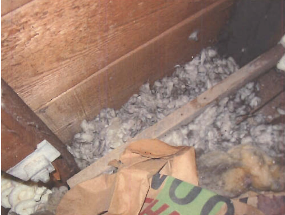
Photo 57: Manotick, Balloon Framing Stud Space
