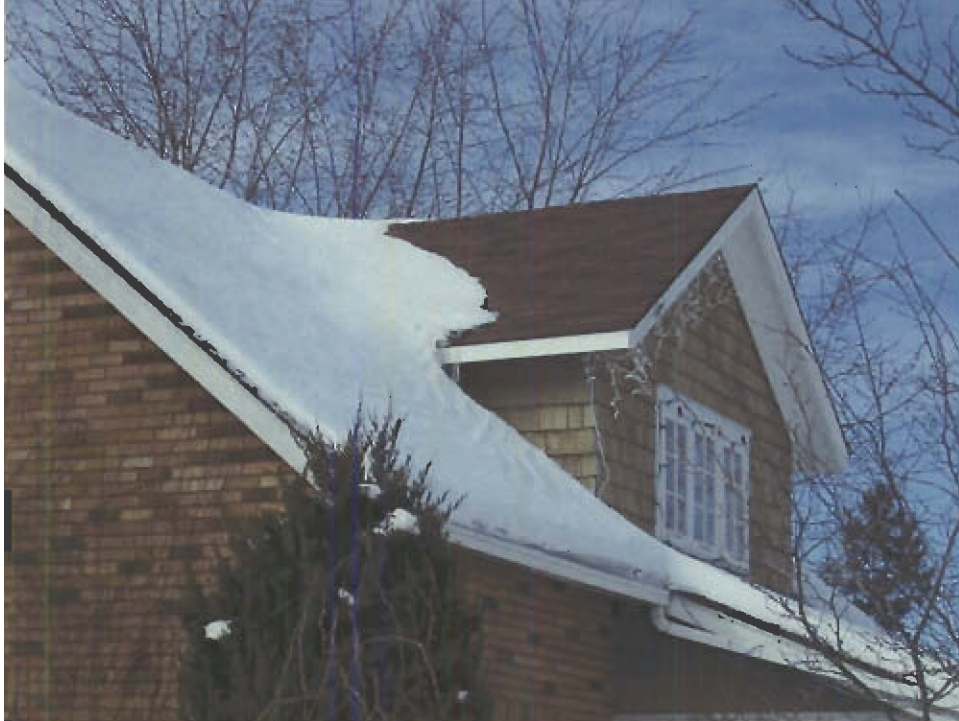
Photo 61: Manotick, Post Repair Snow Cover - Back
