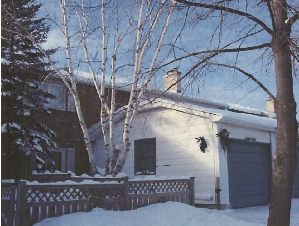
Photo 23: Site 2, Unrepaired Units, January 20, 2004
