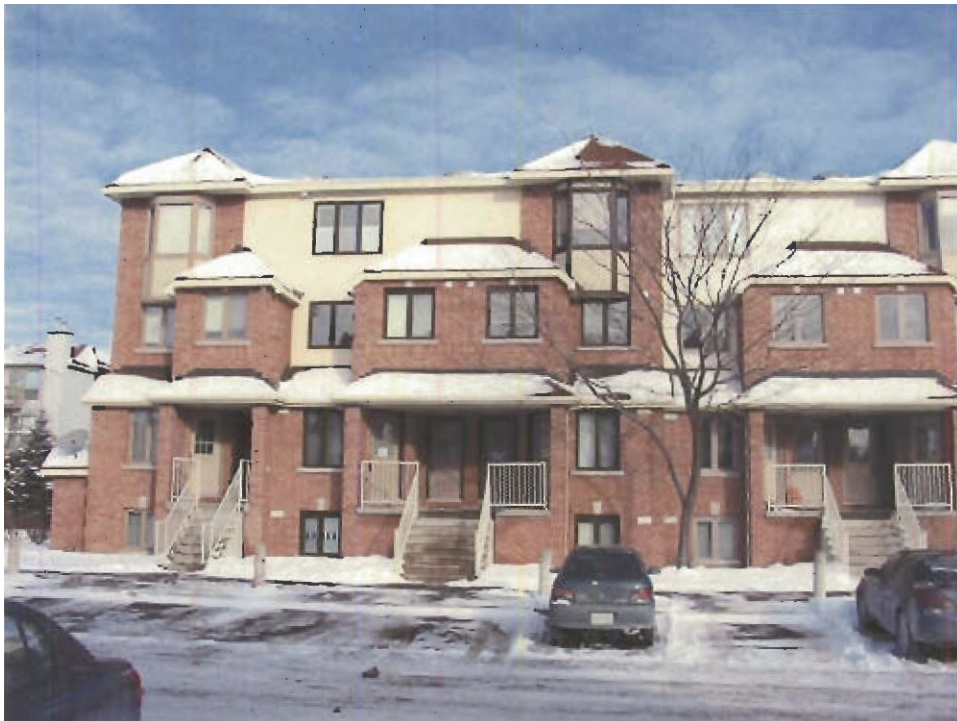
Photo 48: Site 4, Unrepaired Unit (front), January 20, 2004
