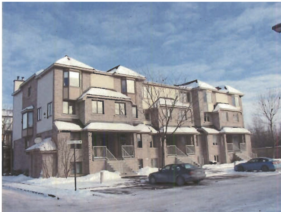
Photo 46: Site 4, Repaired Unit (front), January 20, 2004
