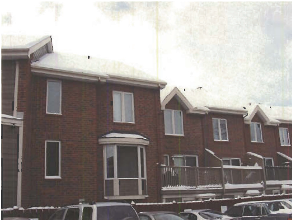
Photo 38: Site 3, Unrepaired Unit (front), January 20, 2004
