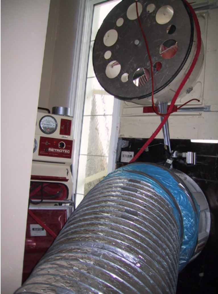
Figure 6: Flex Duct Configuration for Balanced Test
