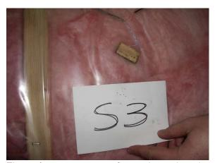
The moisture content wafer on the outboard side of the polyethylene shows mold growth; Delmhorst measurements of the wafer were at 19%.
