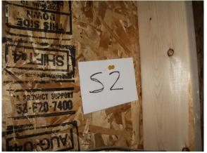
Stud on RH of center bay; no discernable damage to sheathing or framing
