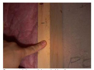
Brown staining at inboard side of upper portion of left-hand test bay stud
