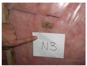
The moisture content wafer at the polyethylene showed mold growth.
