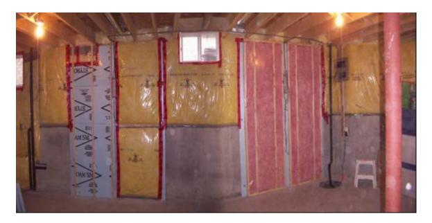
Figure 1.2: Basement walls under construction. Prior to gypsum board installation. From Left to right, XPS, Roll Batt, Stud w/ Poly, Stud w/o Poly.
