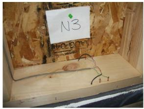
Sill plate showed no evidence of condensation rundown or mold growth.
