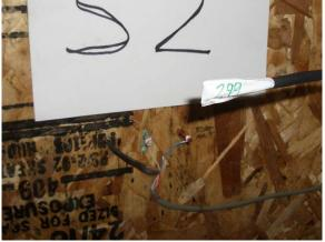
Close-up of the moisture content pins in the sheathing, showing surface corrosion at one of the pins.
