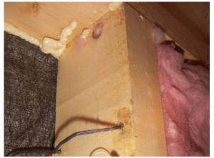
Brown staining at inboard side of upper portion of right-hand test bay stud
