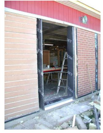
Figure 1.2: Opening details for removable panels
