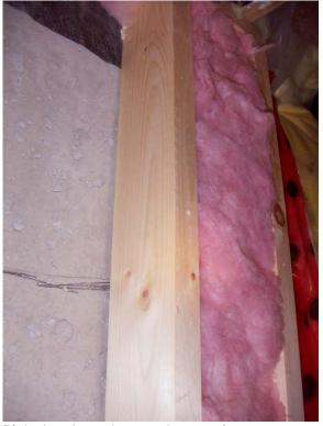
Right hand test bay stud; no moisture evidence seen. The remainder of the frame also showed no evidence of moisture damage.
