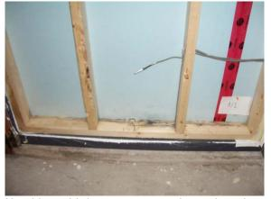
Notable mold damage seen at the outboard side of the sill plate, consistently across the width of the wall.
