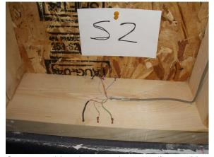
Center stud bay bottom plate; no discernable damage or water staining from rundown.
