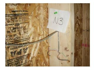
Stud showed no evidence of mold growth; sheathing showed no moisture damage.
