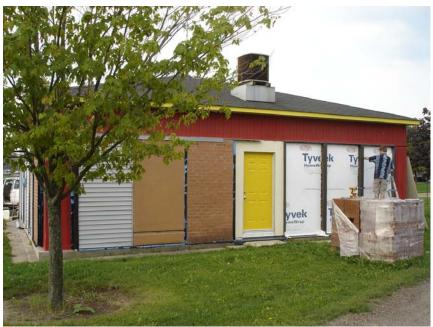
Figure 1.3: South Elevation of BEGHut. Exterior view, SBPO installed. Walls from left to right are Poly, No Poly and XPS
