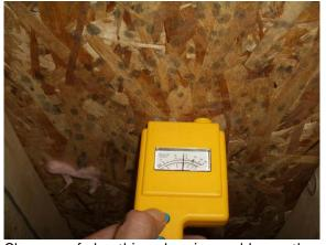
Close up of sheathing showing mold growth, as well as fiberglass adhered to OSB sheathing. There was noticeable grain/flake raising or thickness swelling of the OSB; a straightedge held against the sheathing reveals daylight
