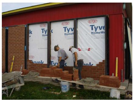
Figure 1.4: South Elevation of BEGHut. Exterior view, bricks being laid.
