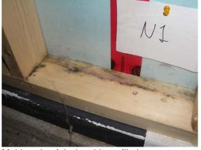
Mold at the right-hand bay sill plate; water wicked under stud at the joint between stud and sill plate. Fiberglass was adhered to sill plate by the mold growth.
