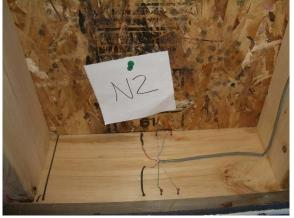
Mold on sheathing, and evidence of water rundown on the outboard side of sill plate. However, framing showed only traces of visible mold, only on sill plate.
