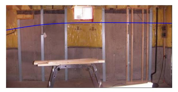
Figure 1.1: Basement walls under construction. Concrete foundation wall visible. Blue line indicates exterior grade level.
