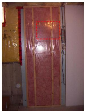
The only notable observation during initial opening was the mold growth on the upper moisture content wafer, located at the grade/below grade intersection, on the interior side.
