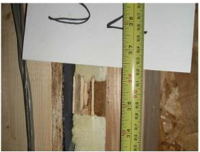
A pair of stains on the back of the drywall caused questions at first; they were both located approximately 36" off of the bottom of the wall. Measurement s showed that they matched up exactly with the cedar shims used to hold the walls in place. These stains are likely extractives from the end grain of the shim spacers.
