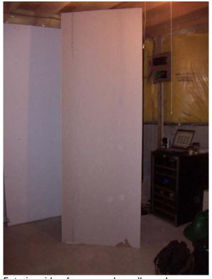
Exterior side of gypsum drywall; no damage or evidence of moisture accumulation. Circles visible in image are dust/flash photographic artifacts.
