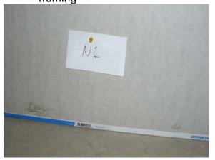
The back of the drywall showed some water staining, matching the locations where the studs butt into the sill plate.
