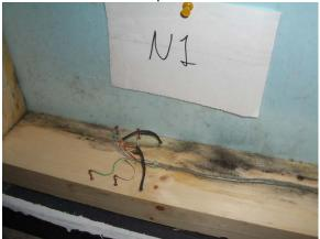
Greatest mold growth at center bay sill plate. Black mold evident on sheathing.
