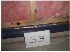
Mold damage was visible on the inboard side of much of the framing, especially at the bottom plate, with some visible condensation on the polyethylene.
