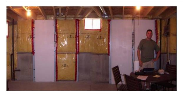
Figure 1.3: Basement walls Completed. Painted gypsum board in place.
