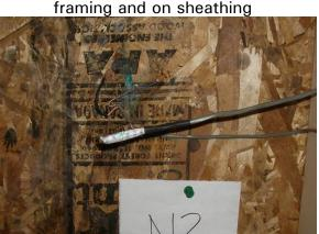
The sheathing showed well-distributed mold; the moisture content pin showed corrosion sufficiently advanced to warrant replacement.
