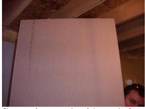
Close-up of upper portion of the exterior face of gypsum drywall; no moisture damage seen.
