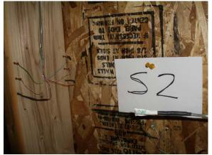
Mid-height monitoring area; no discernable damage to sheathing or framing
