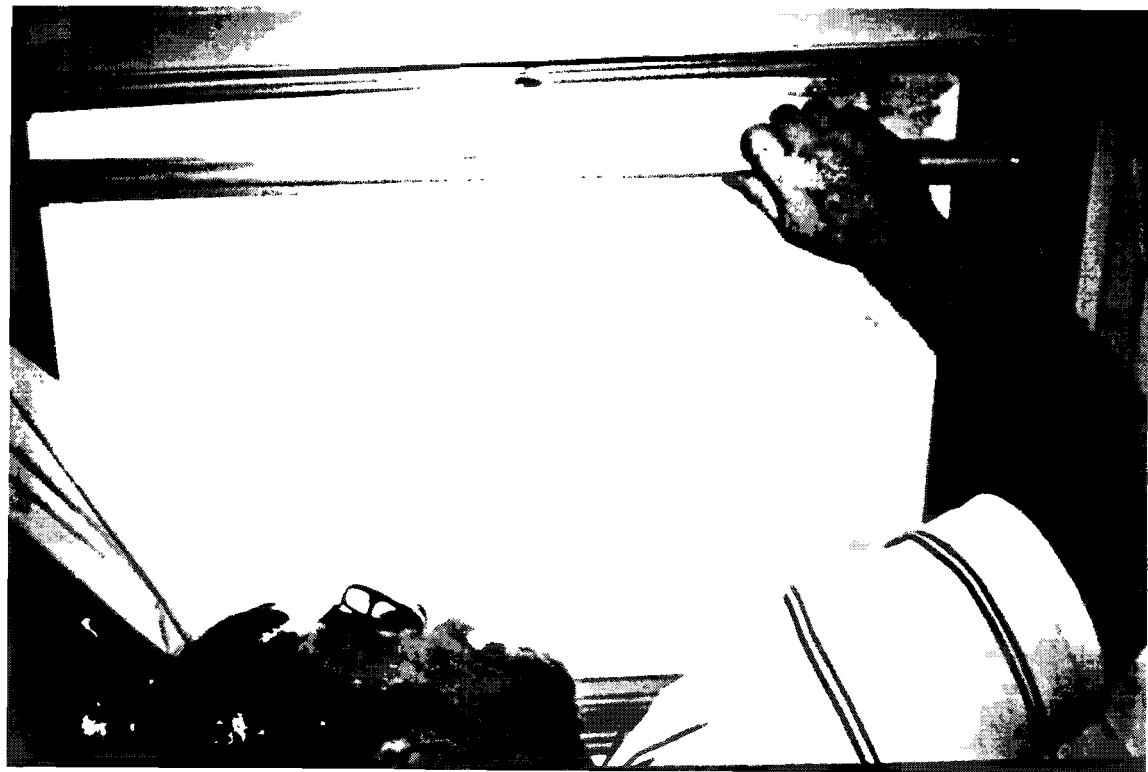
Window sashes were removed, the weatherstripping was replaced then the sashes were reinstalled.
