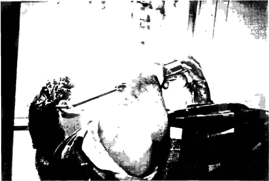
Air sealing work included window trim caulking.
