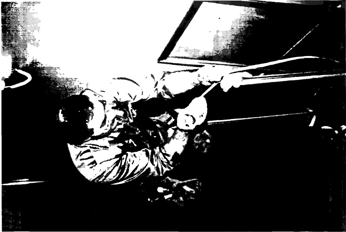
Window sashes were removed, the weatherstripping was replaced then the sashes were reinstalled.
