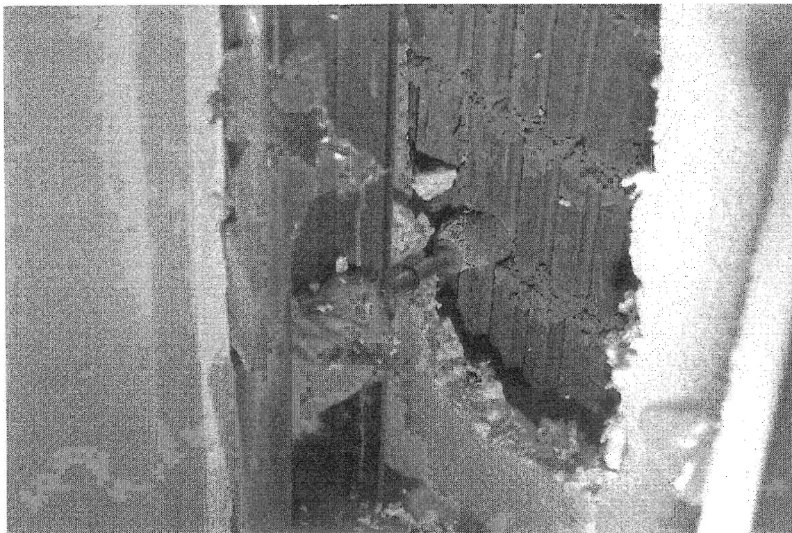
Photo 16 - Interior View of EXT2 - Cintec Repair System
