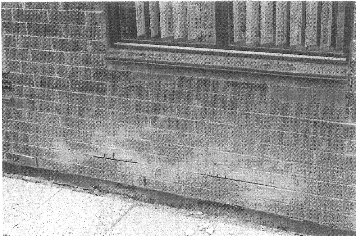
Photo 4 - Location of Studs by Saw-Cutting the Mortar Joint
