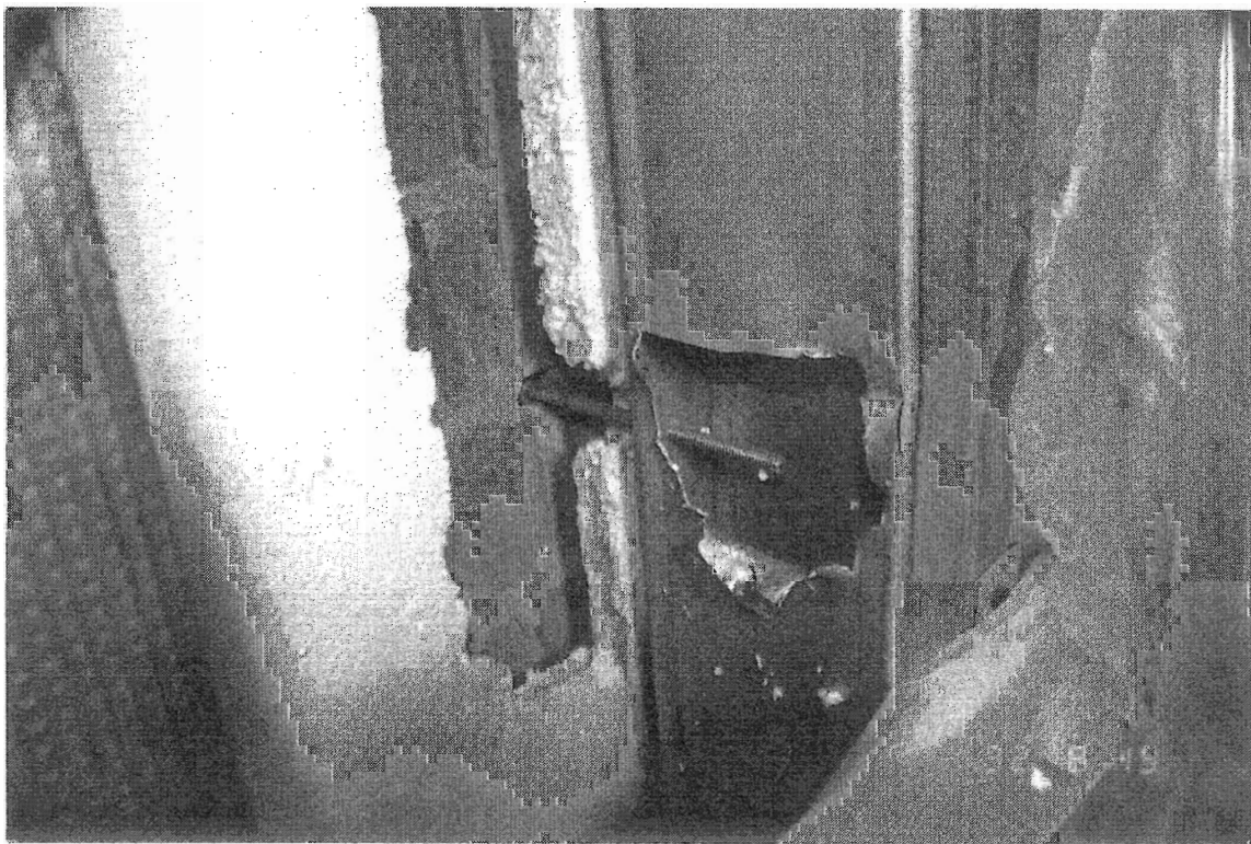
Photo 22 - Interior View of Repair EXT5 Connection to Steel Stud
