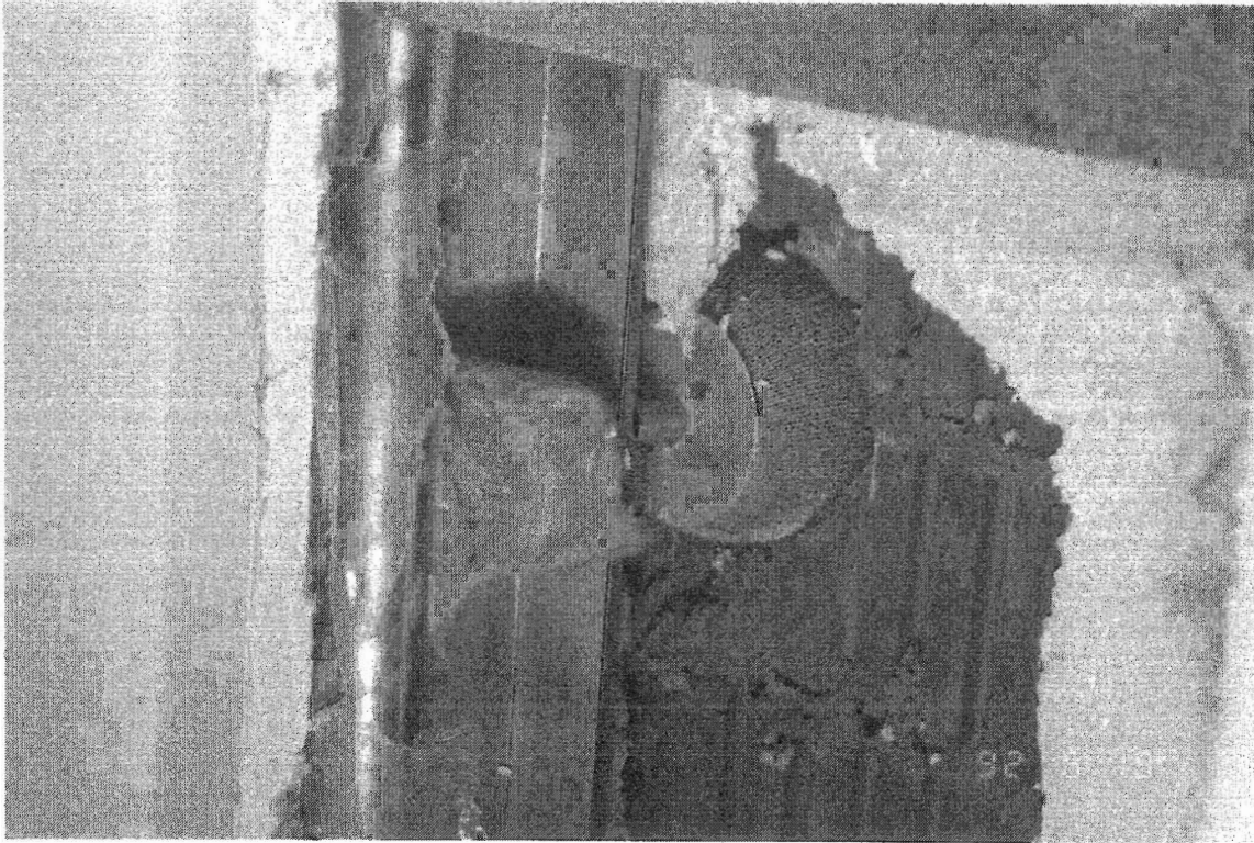
Photo 13 - Interior View of EXT1 - Cintec Repair
