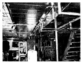
Picture, <u>H3,006.jpg</u>, shows the tapered end on the return-air trunk, used by the contractor to extend the return-air far enough to pick up the floor return-air grille from the living room. The taper was also necessary to enable continuation of the 10"x8" supply trunk.
