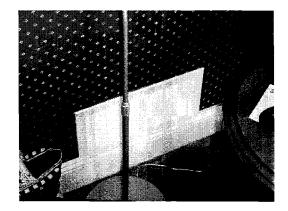
Picture, <u>H2,013.jpg</u>, shows plate opening at top of stud space, alignment of studs and joists does not always allow for a full stud pass to be open to a single joist space. Insulation required for the radiant heating panels had to be removed from those cavities used for passage of return air and cavities had to be sealed from neighbouring spaces. Insulation was still required above that portion of the ceiling containing radiant ceiling panels.
