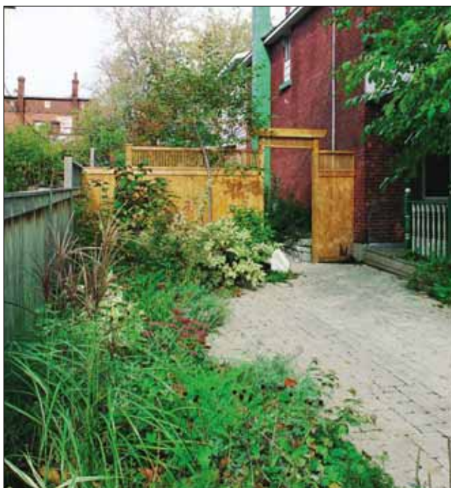
Figure 7 To reduce runoff and beautify the property, the homeowners reduced the size of their driveway by more than 60 per cent by replacing it with plantings. They changed the material on the remaining driveway from asphalt to precast concrete pavers.
