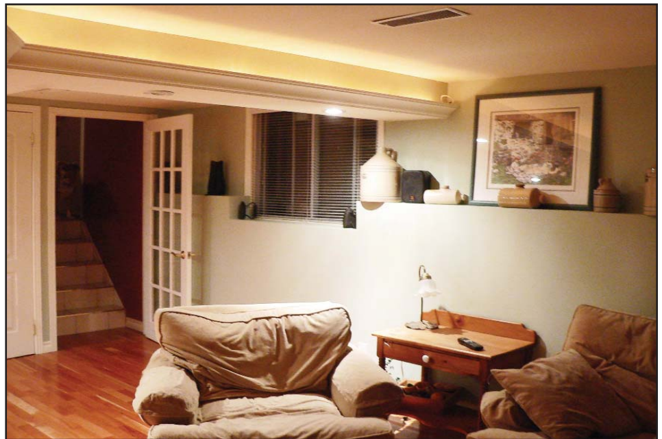
Figure 5 Heating plenum disguised as a lighting fixture
