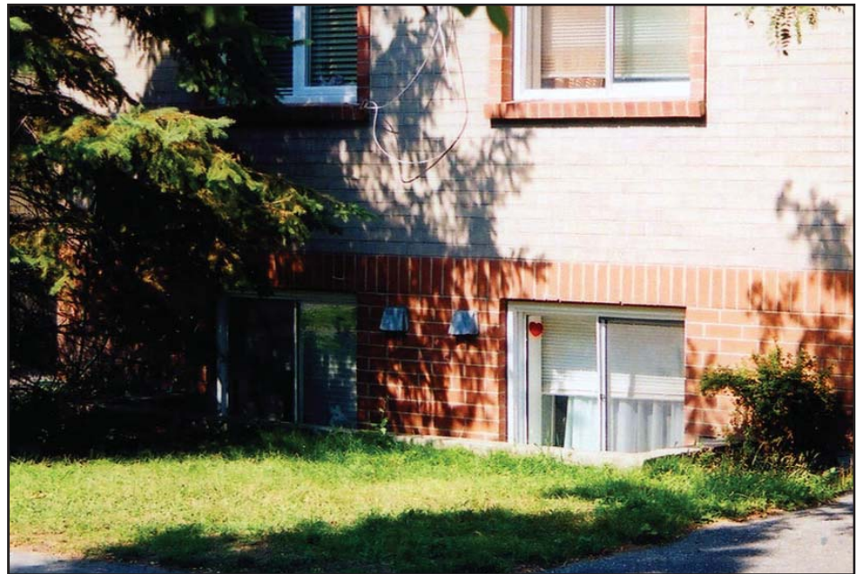
Figure 6 Large wells permit big basement windows, improve natural light and ventilation and may facilitate exiting
