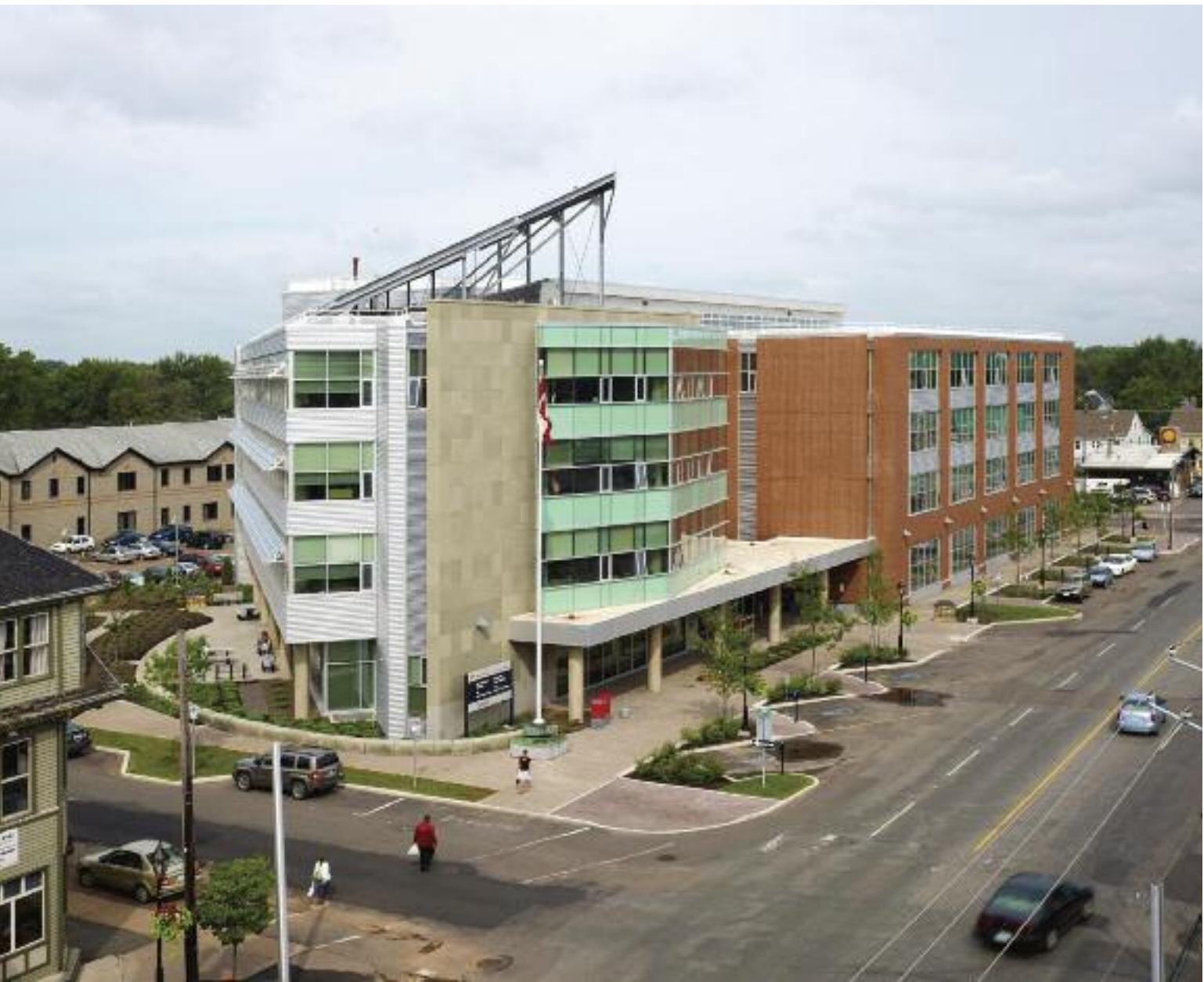
Jean Cantfield Building - Charlottetown, Prince Edward Island, Crown-Owned (application pending for LEED Gold certification)
