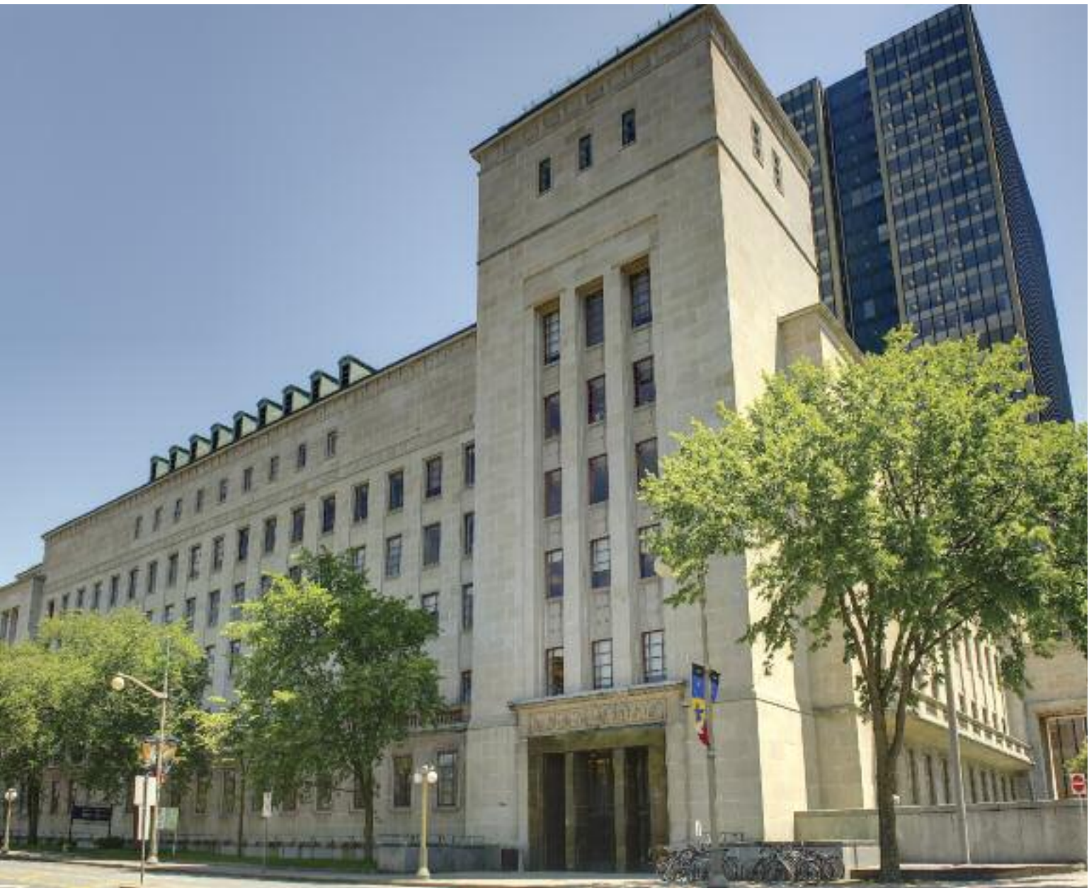
East Memorial Building – 284 Wellington Street, Ottawa, Ontario, Crown-Owned
