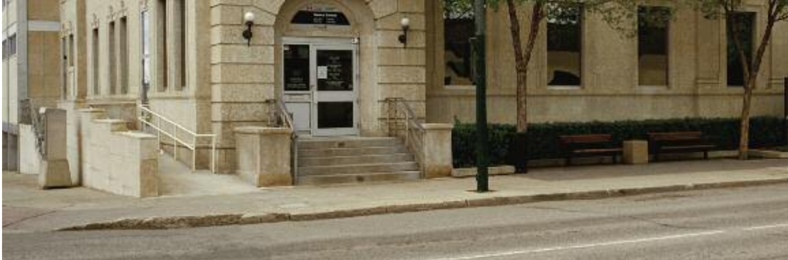
Ramp at the Brandon Federal Building - 1039 Princess Avenue, Brandon, Manitoba, Crown-Owned.
