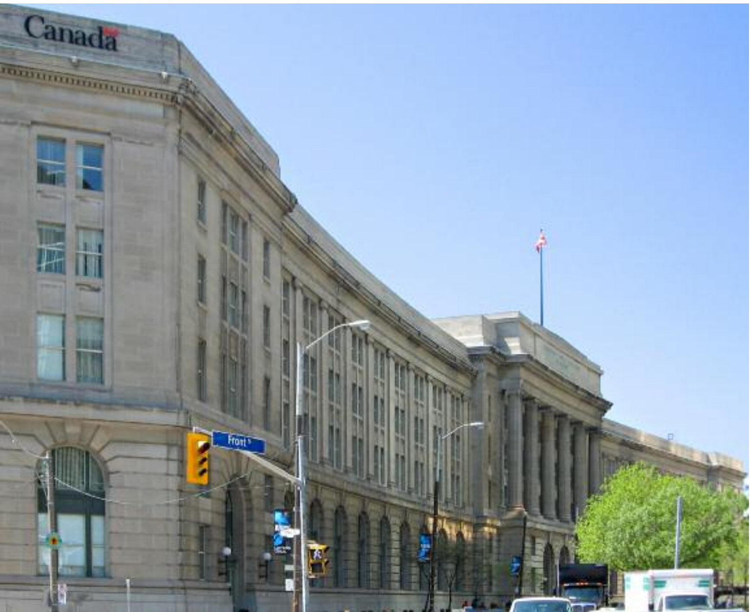
Dominion Public Building - 1 Front Street, West, Toronto Ontario, Crown-Owned
