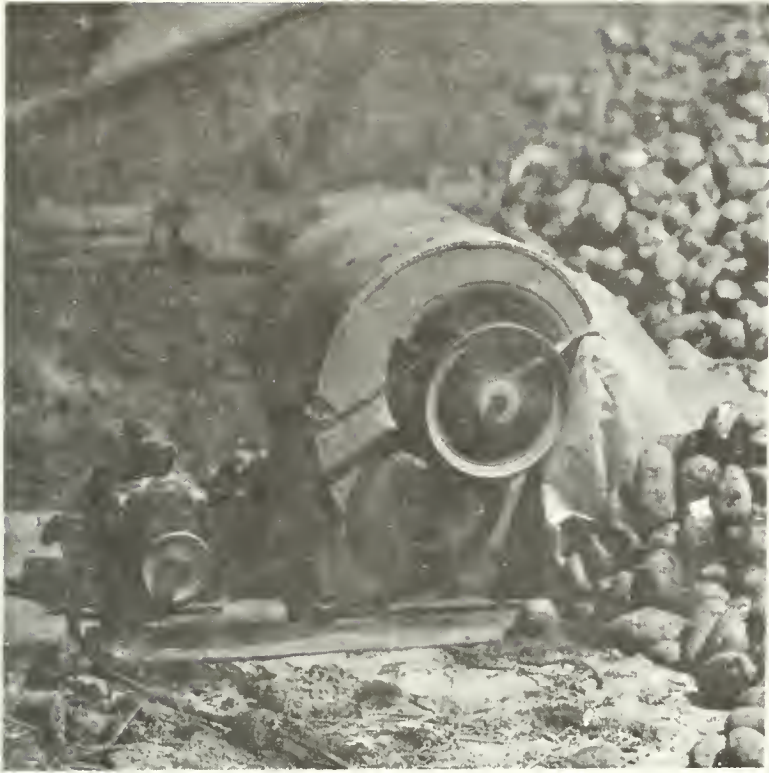
Fig. 24 Portable ventilation fan unit attached to duct opening.
