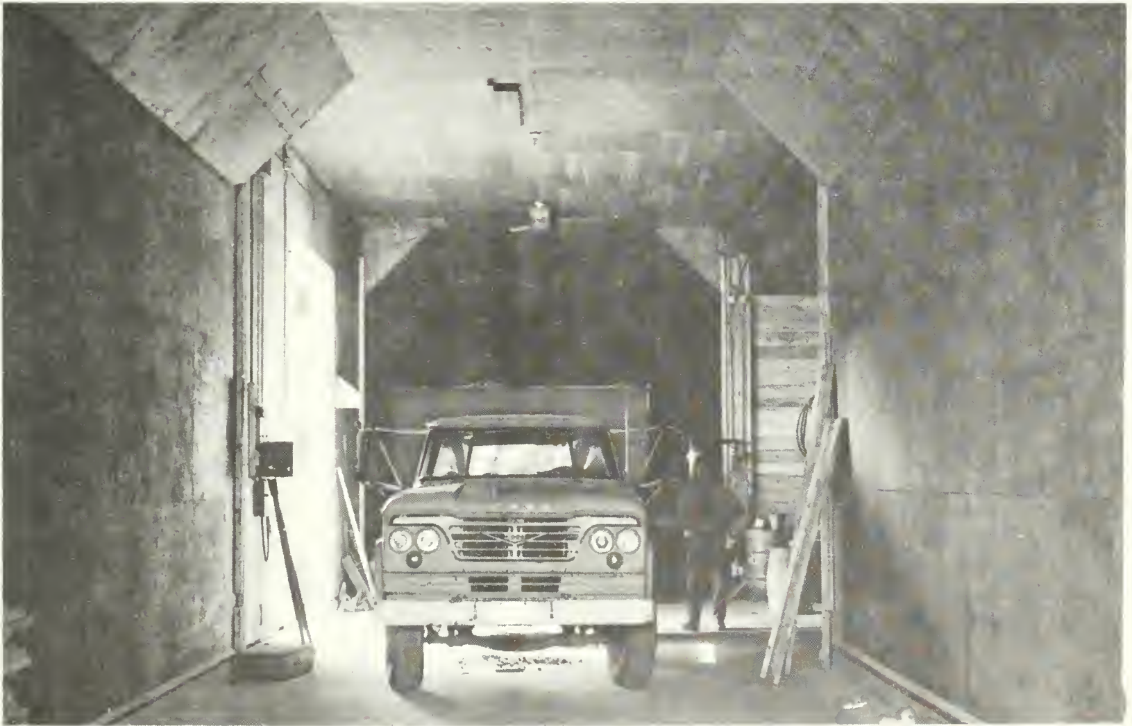
Fig. 26 Air delivery system using wall and bin partition spaces as air ducts.
