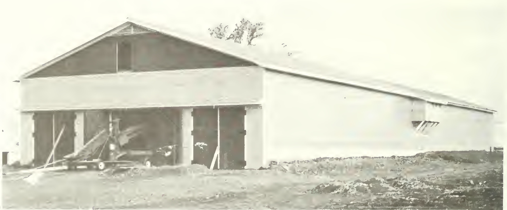
Fig. 1 Potato storage with wood frame construction, steel cladding and trussed rafters.
