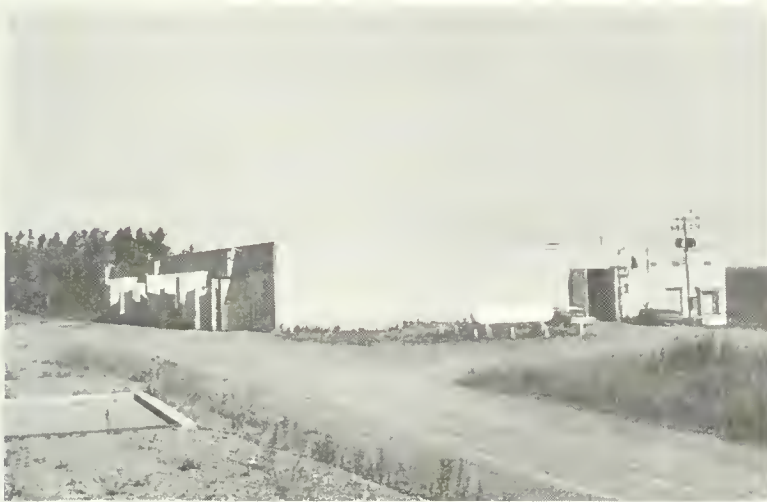
Fig. 5 Large steel frame storage.
