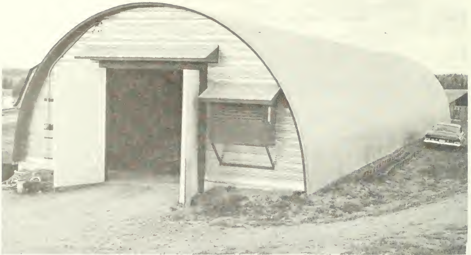
Fig. 3 Arch roof potato storage.
