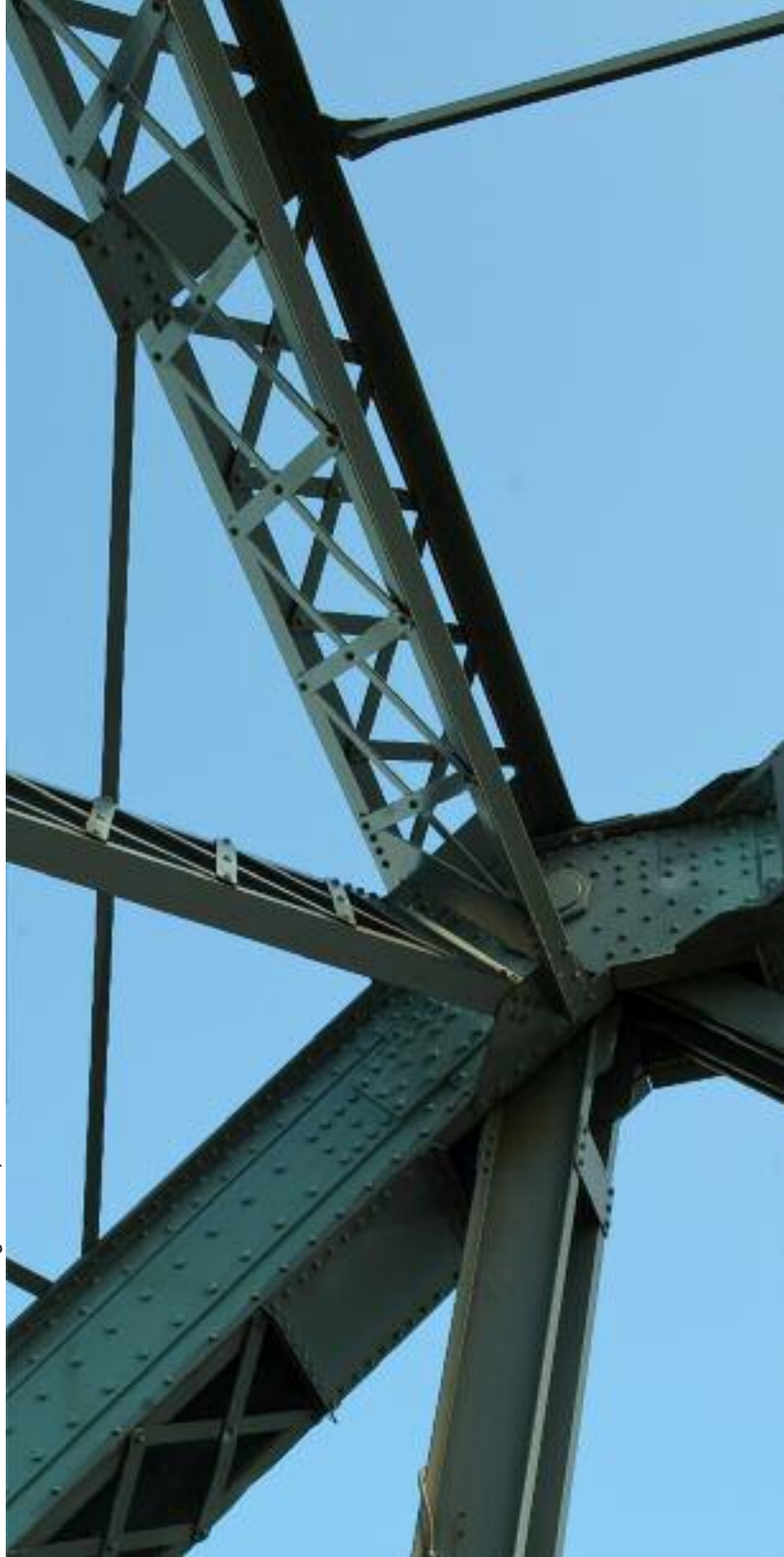
Alexandra Bridge—Detail, Crown-owned
