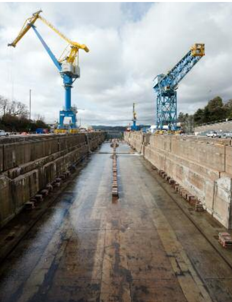
Esquimalt Graving Dock—825 Admirals Road, Esquimalt, British Columbia, Crown-owned
