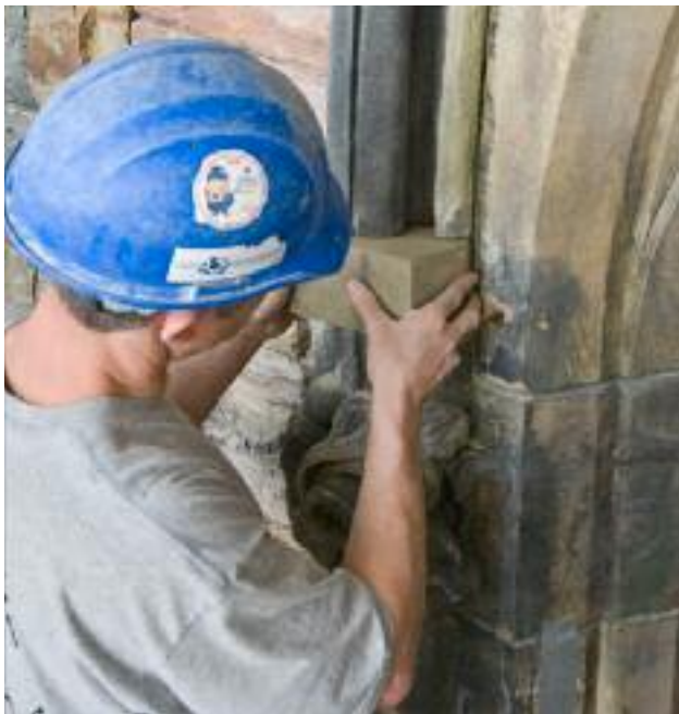
Interior masonry work—Parliament Hill, Ottawa, Ontario
