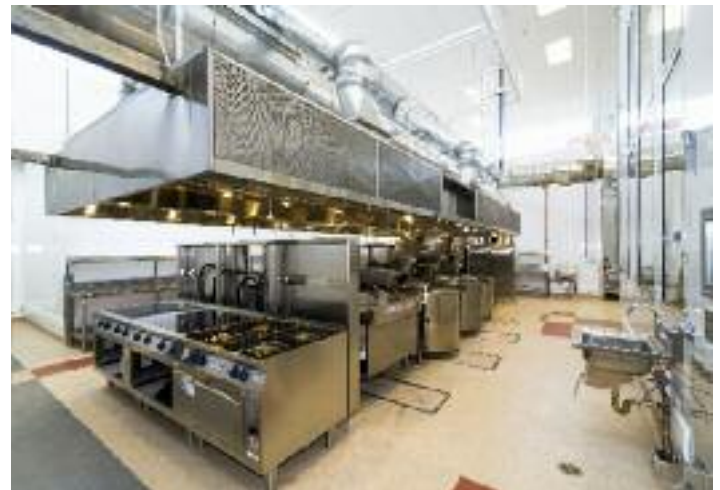
Food Production Facility—1170 Algoma Road, Ottawa, Ontario, Crown-owned
