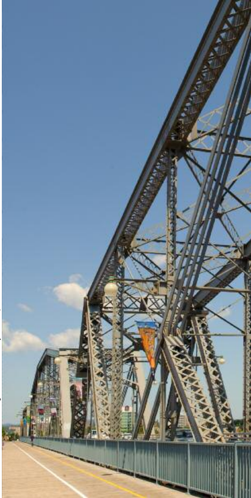
Alexandra Bridge—Pedestrian and bicycle access, Crown-owned
