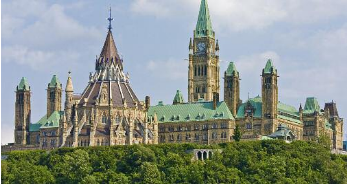
Centre Block—111 Wellington Street, Ottawa, Ontario, Crown-owned
