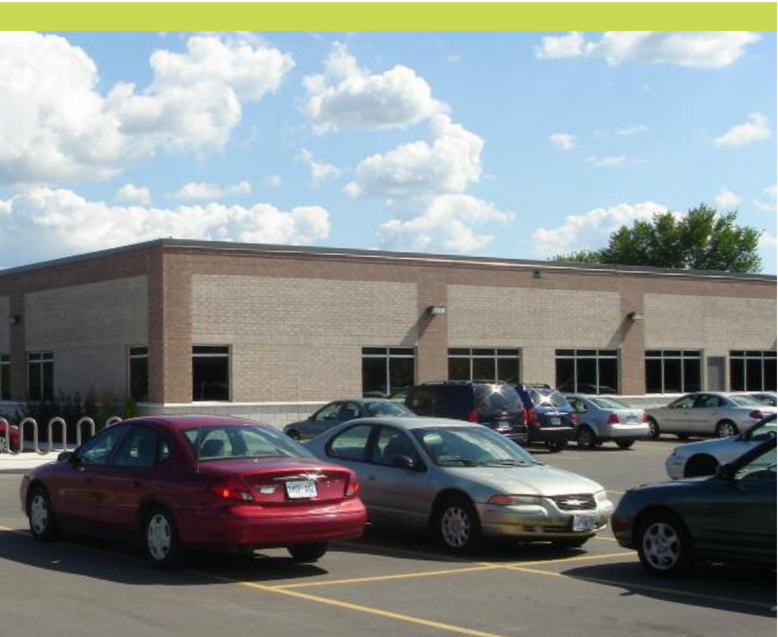
Government of Canada Building—551 Campbell Street, Cornwall, Ontario, leased
