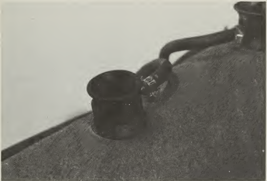
Fig. 16 Close-up of a grommet assembly for an air-assisted sprayer.
