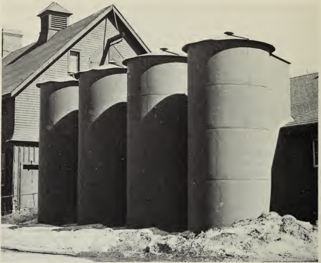
Bank of four insulated plywood silos for storing experimental silage at the Animal Research Institute, Ottawa.
