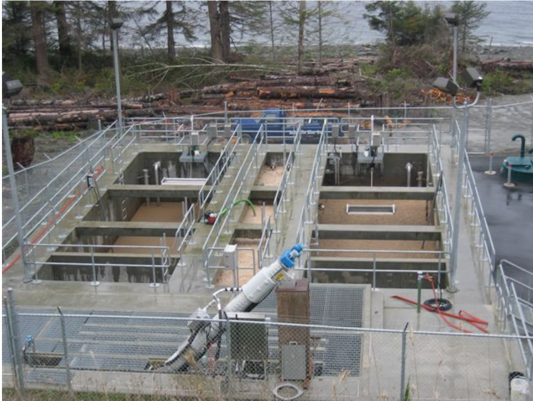
Typical Mechanical Wastewater Treatment Plant
