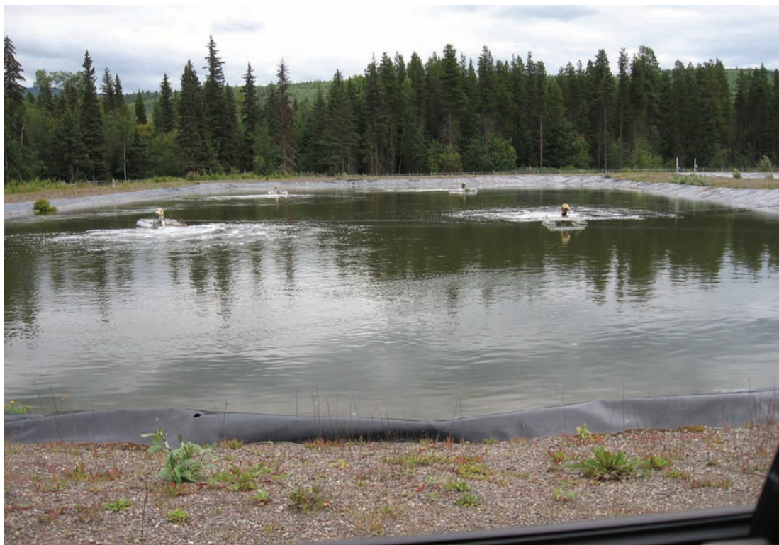
Lagoon Surface Aerators
