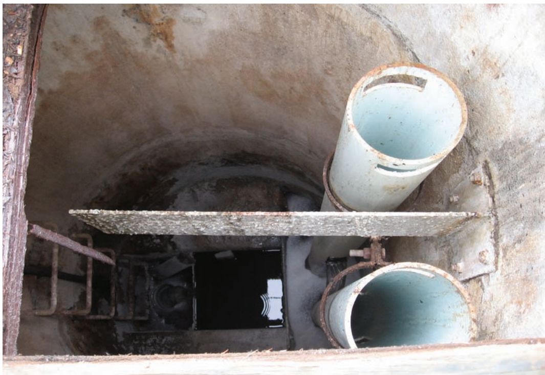
Lagoon Outlet Weir
