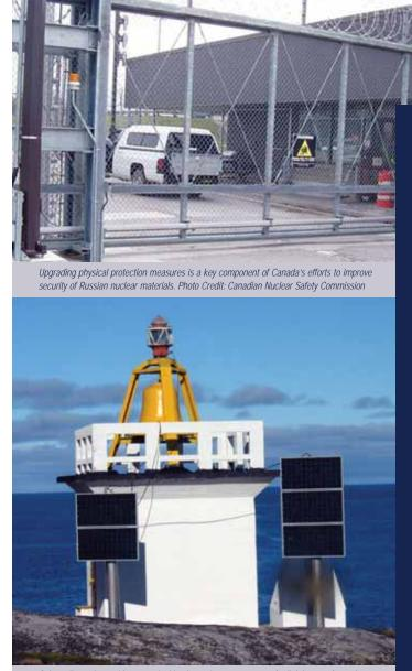
Solar cell panels provide a sustainable alternative power source for lighthouses formerly powered by highly radioactive material. Photo Credit: County Governor of Finnmark (Norway)
