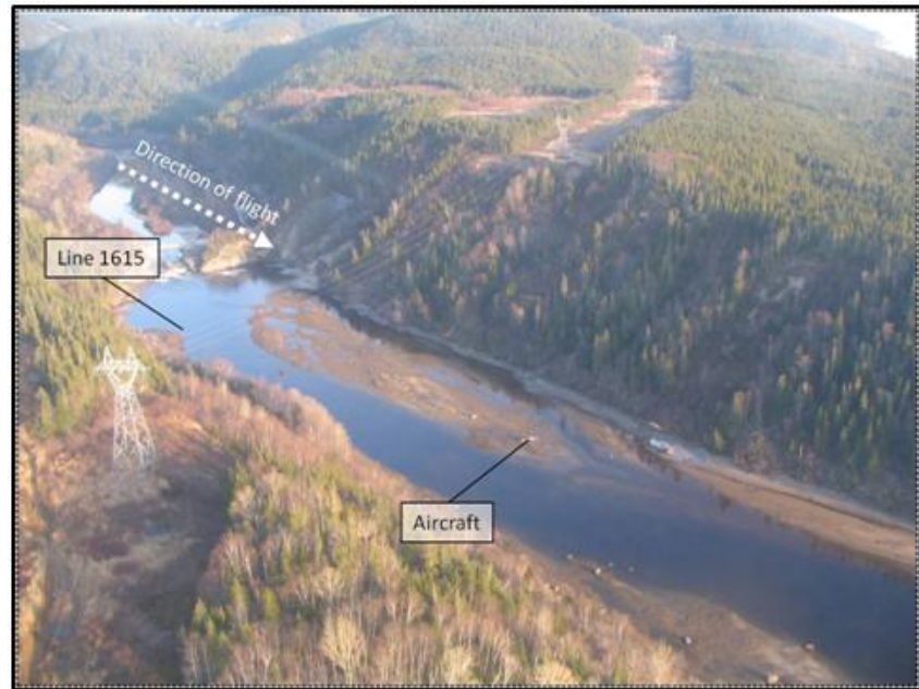
Photo 2. Aerial view of accident site
