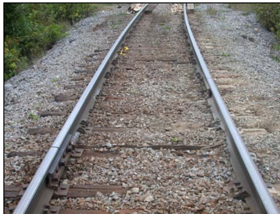
Photo 3. View looking northward showing location of rail joints
