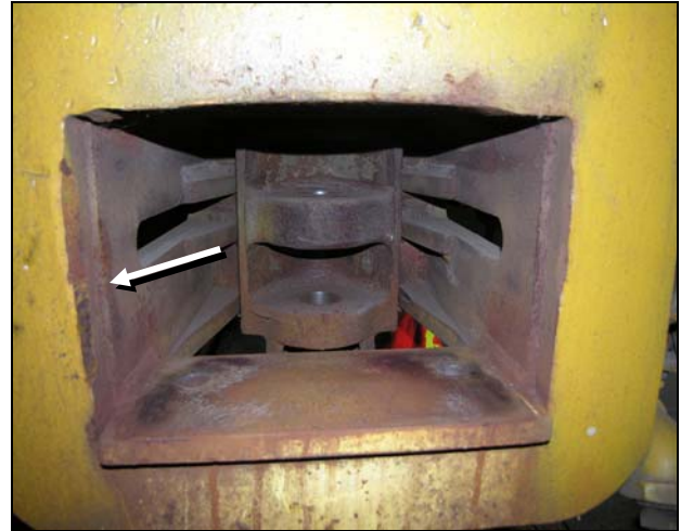
Photo 2b. Impact marks on the end sill opening
