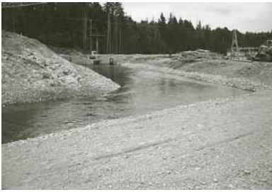
A proposed development project has barriers at the riverbanks to prevent erosion of soil, which could be carried downstream to salmon spawning areas.
