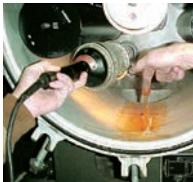
Figure 2. Apple Jelly Found in a Horizontal Filter Vessel
