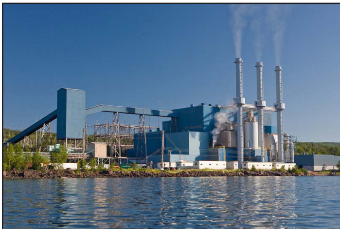
Taconite Harbor Energy Center
