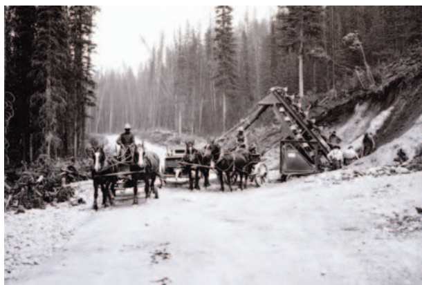
Road construction at Marble Canyon, Banff-Windermere Highway Kootenay NP of Canada (B.C.) © Parks Canada PHOTO: Parks Canada
