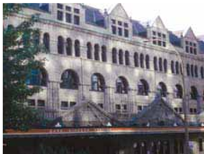
New Roman style building constructed in 1888-1889. Windsor Station (CP) National Historic Site of Canada (QC) © Parks Canada, PHOTO: C. Rodriguez
