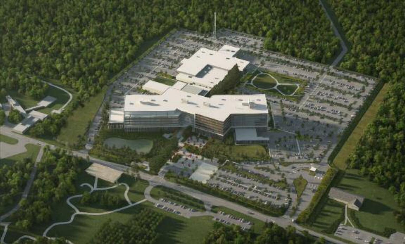
Aerial View of RCMP E Division Headquarters—14200 Green Timbers Way, Surrey, British-Columbia, Lease Purchase
