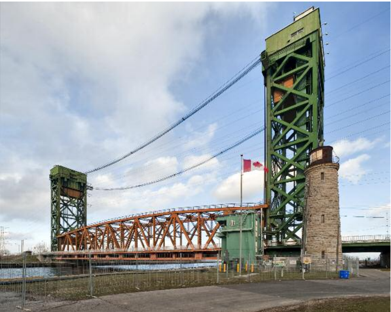
Burlington Lift Bridge—Hamilton, Ontario
