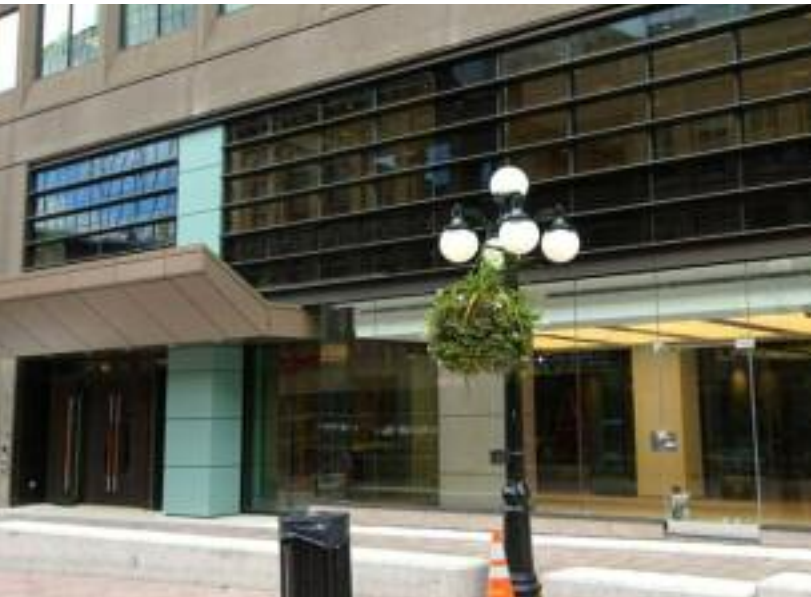
Entrance to the newly renovated La Promenade Building, Sparks Street, Ottawa, Ontario
