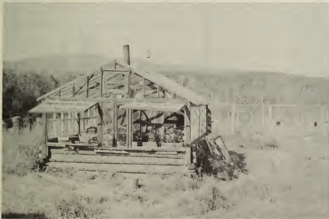
Figure 10 - A greenhouse made of logs, old sash windows and other materials on hand at Old Crow, Y.T. 72 miles north of the Arctic Circle.
