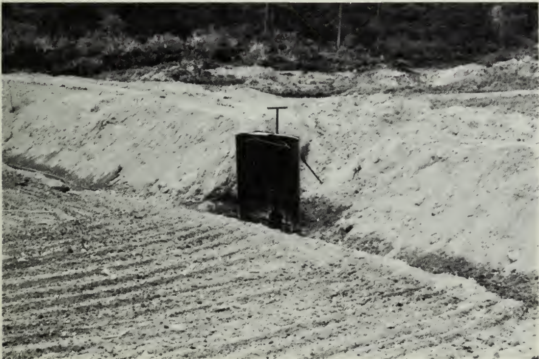
FIGURE 6 The bulkhead was made by cutting an oil storage tank in two. The valve, turned from above, regulates the water level for harvesting.
