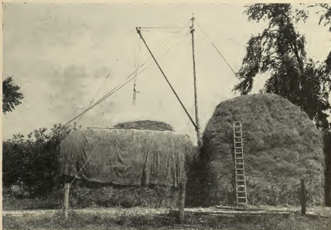
With the mast and boom staker four stacks can be built at each setting of the staker.
