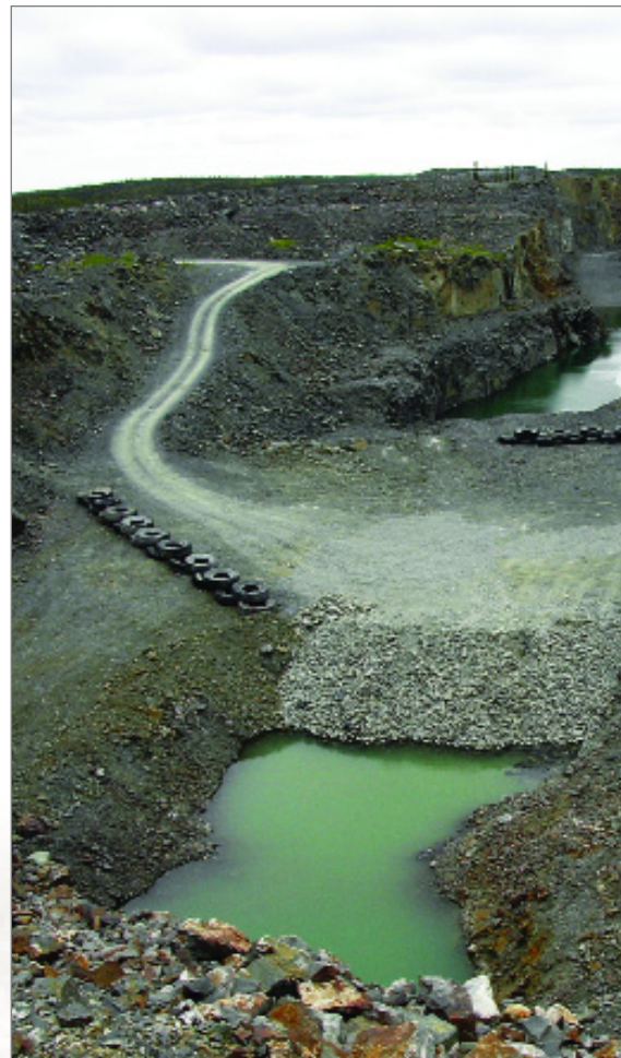
Medium-sized materials too large for the LTU were placed in the Zone 2.5 Pit.
