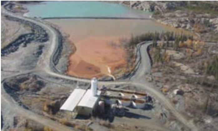
An aerial overview of the Effluent Treatment Plant, polishing and settling ponds at Giant Mine
