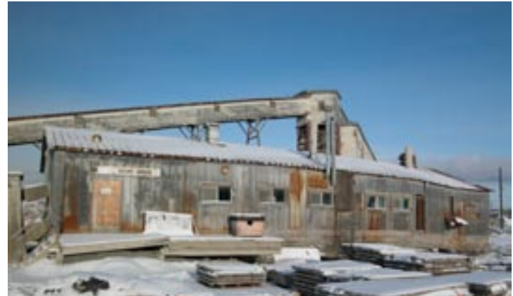
The Assay Office at Giant Mine is one of more than 100 buildings on site scheduled for demolition
