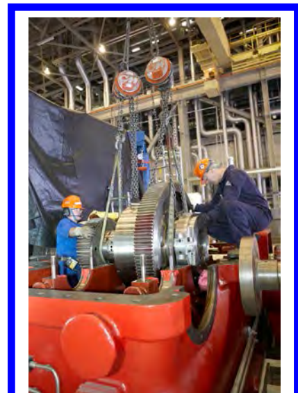
Outage maintenance work at Darlington.
