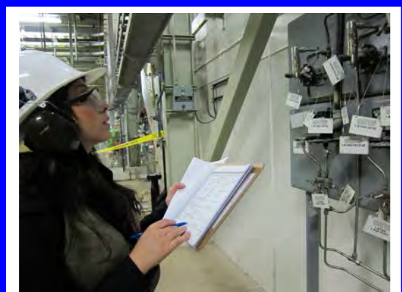
A CNSC site staff member inspects an instrument panel at the pumphouse that draws cooling water.
